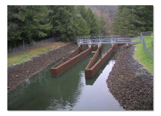
Maintain and operate a tailrace weir designed to increase DO levels above MD water quality standards.
