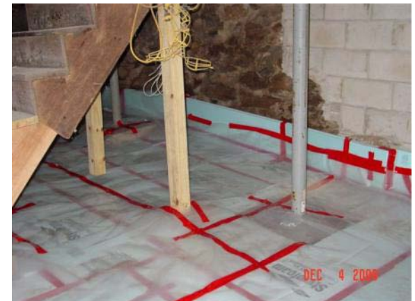
Basement prepared for slab
