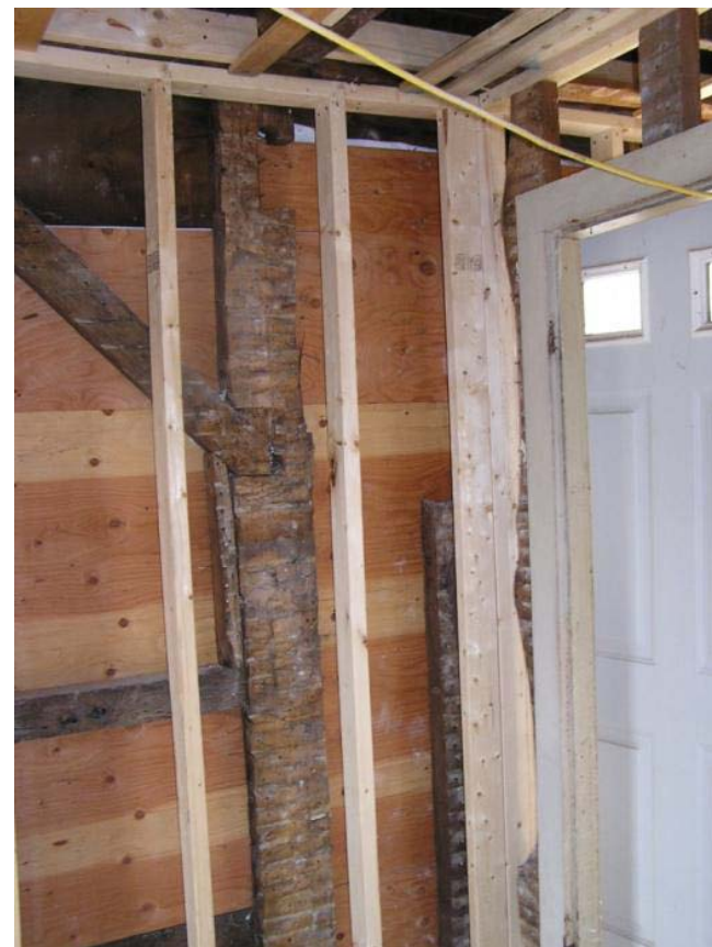
Stud wall constructed to interior
