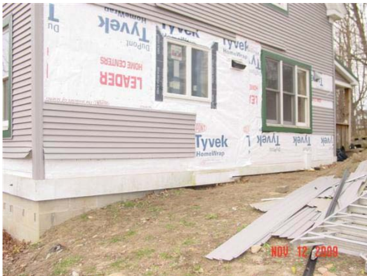
Siding removed to remediate flashing
