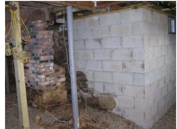
Basement gravel fill and chimney demolition
