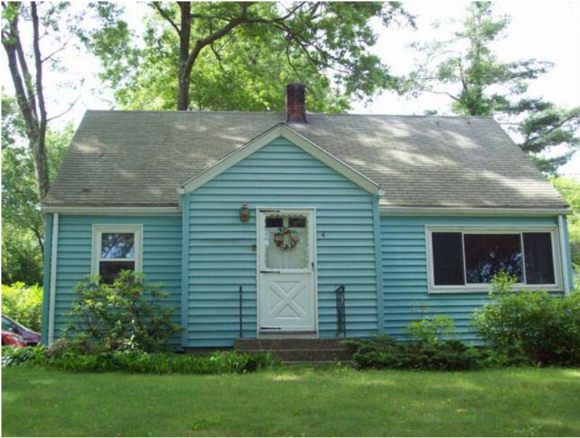
Tweedly residence pre-retrofit
