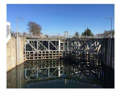
As part of the project, a set of locks were added at the eastern end of the barge canal to allow for a short-cut between the port and the Sacramento River. Because the height of the river can tower some 20 feet over the barge canal at the river's high water mark, the locks were built with a transition height of 21 feet. In honor of Stone's unofficial title as "Father of the Port of Sacramento," the locks were named for him.
