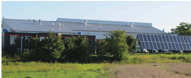
Figure 5.4 FlexHouse and PV installation at RISØ DTU
