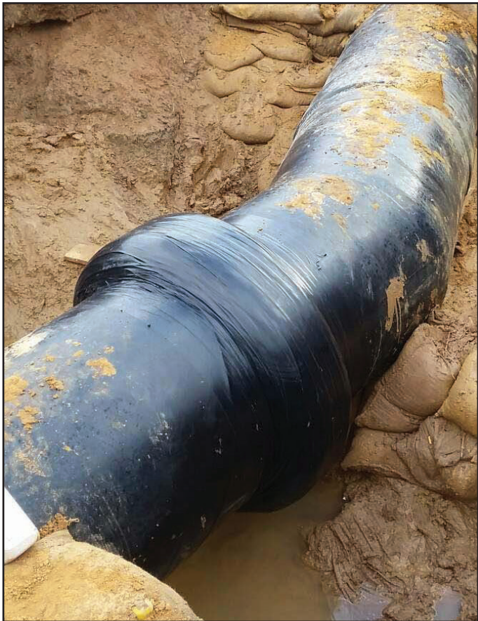
A wrap of Denso PVC SA™ Tape completes the system.
