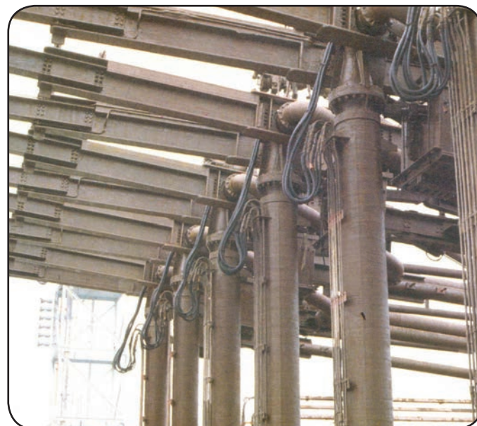
UK - Protecting loading booms at the Esso Milford Haven Refinery, using weatherboard and spiral tape wrapping techniques.
