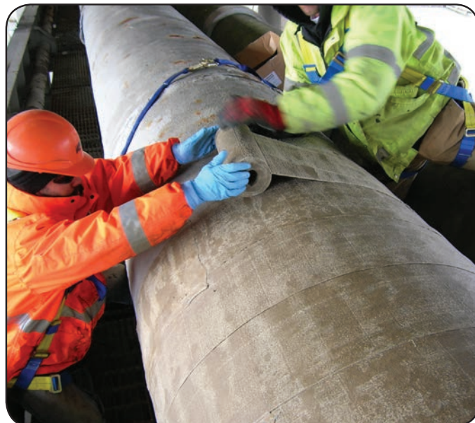
Canada - Protecting a sweating concrete water pipeline in sub zero conditions. Halton Region near Toronto.
