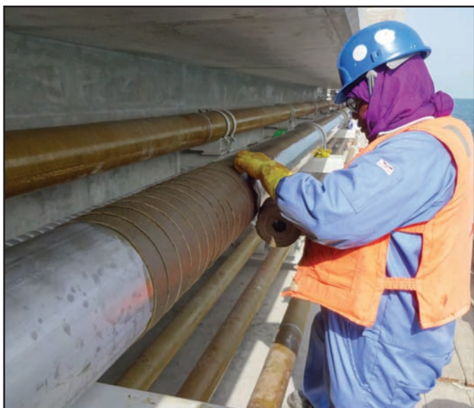
First a coat of Denso Paste™ is followed by a spiral wrap of Densyl™ Petrolatum Tape.
