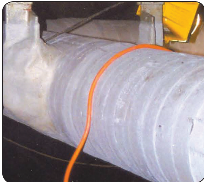
Australia - Protecting United Energy gas pipework and fittings in a confined space under the Spencer Street Bridge in downtown Melbourne.
