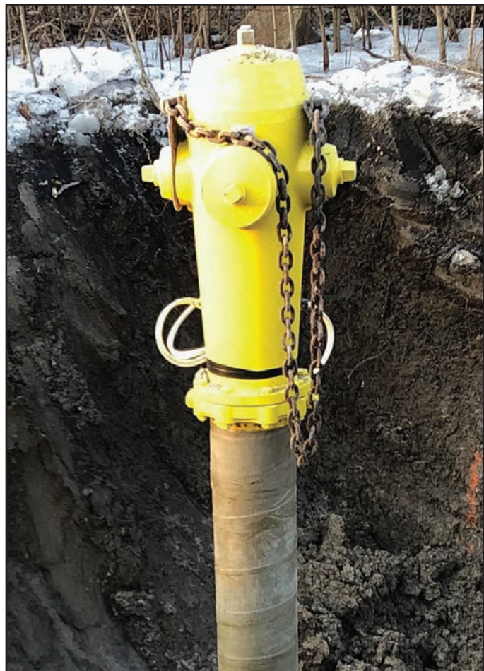
Water hydrant supply pipework protected with the Denso LT™ Petrolatum System.
