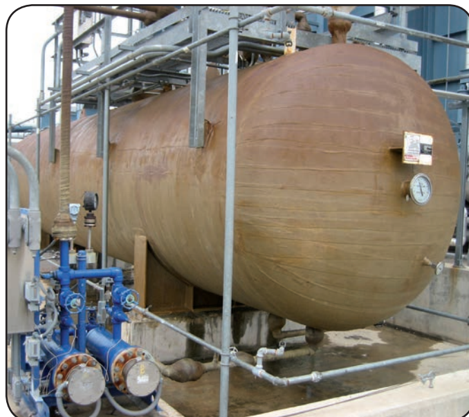
USA - Protecting constantly sweating steel ammonia tanks at the Lower Colorado River Authority (LCRA) Bastrop facility, Texas.
