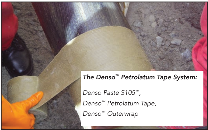
The Denso™ Petrolatum System was applied to protect the pipe.
