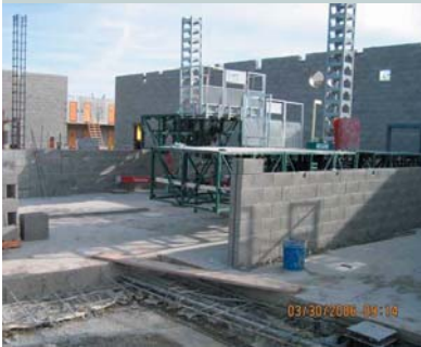
Washington State Penitentiary expansion housing unit
