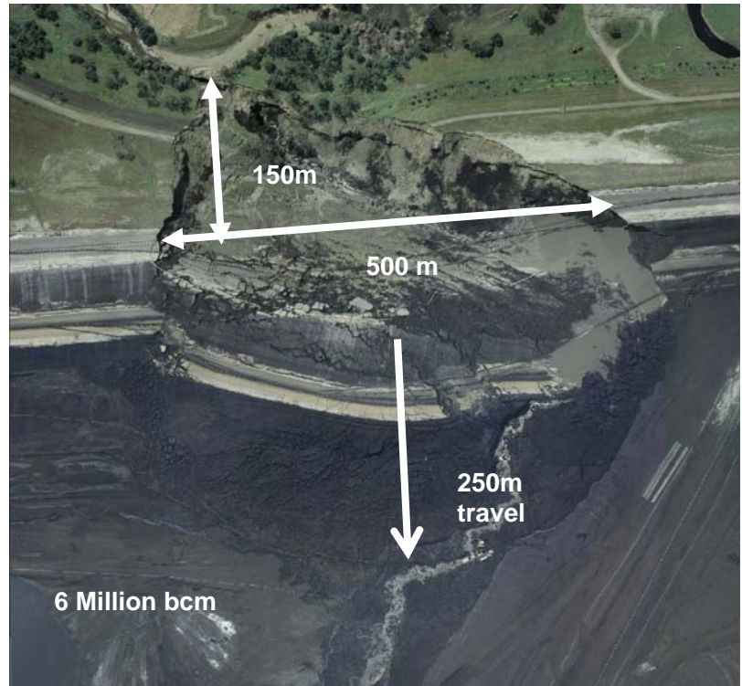
Figure 4.1 Site of mine collapse, indicating scale
