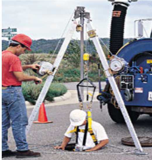
Tripod used for safe entry
