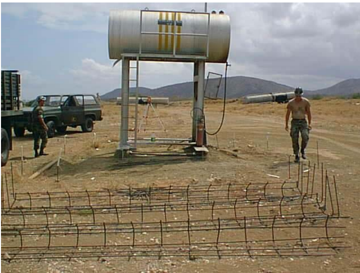
Spill Containment Before
