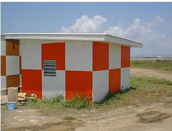
Repairs to VOR Generator Building
