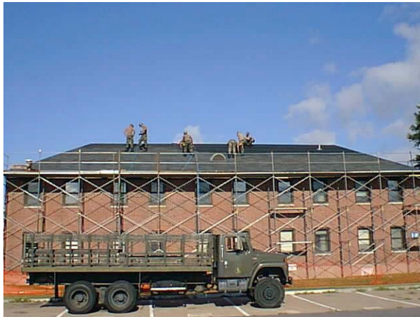
Exterior Repairs in Progress
