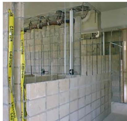
CMU Construction in Head Area
