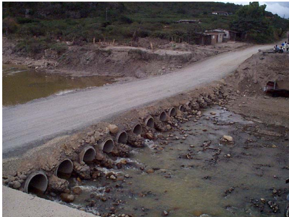
Completed Low Water Culvert Crossing
