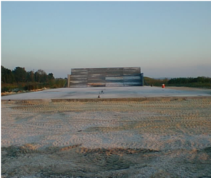
JX7-804: CONSTRUCT NEW TRAINING CENTER
