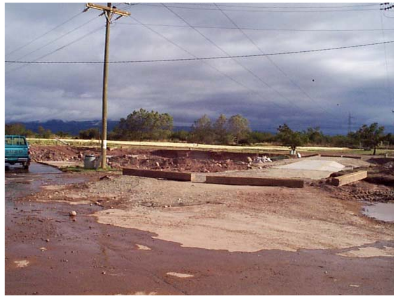
After Tank Removal
