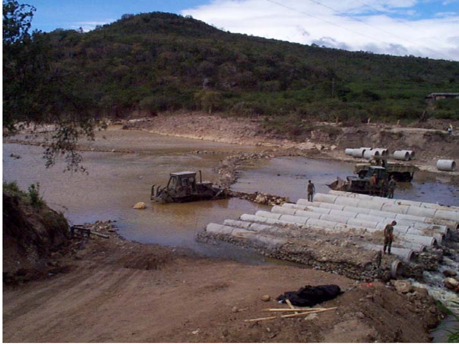
Completed Low Water Culvert Crossing
