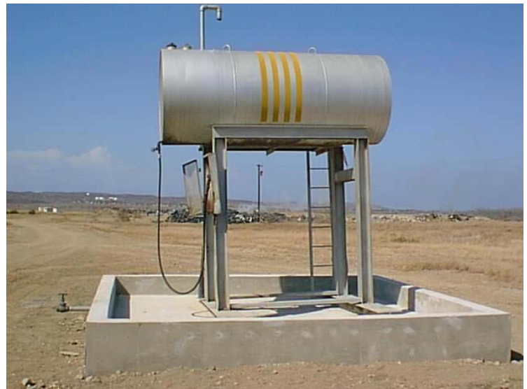
Spill Containment After
