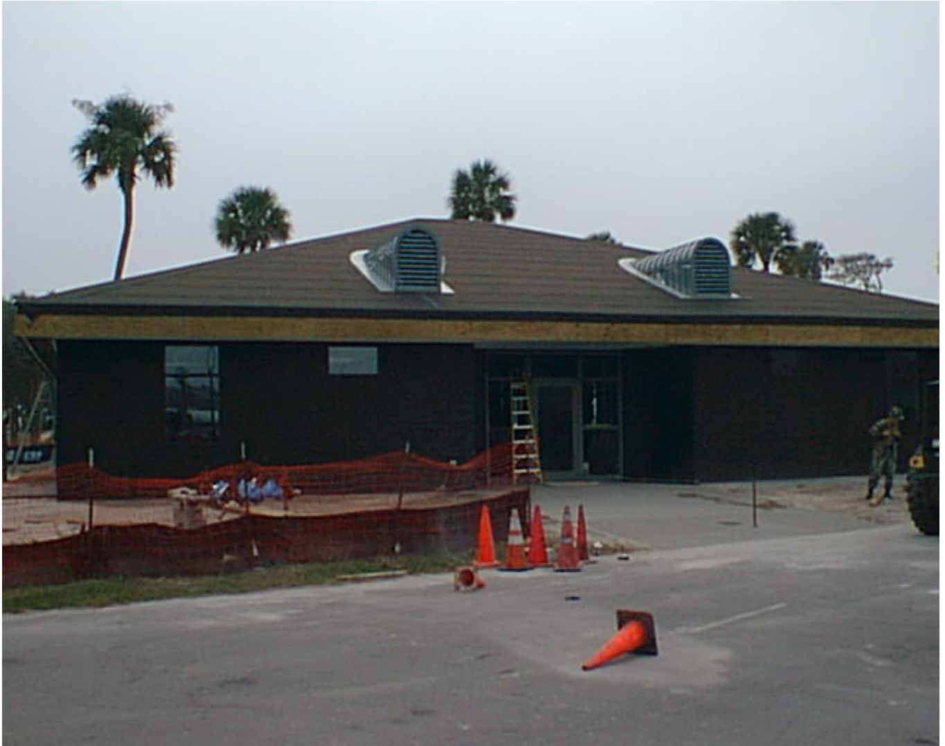
MP8-801 CONSTRUCT DENTAL CLINIC
