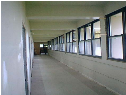
New Interior Finish of Barracks
