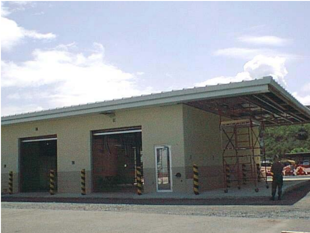
Facility Nearing Completion
