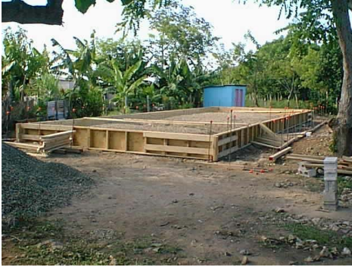
Schoolhouse Under Construction
