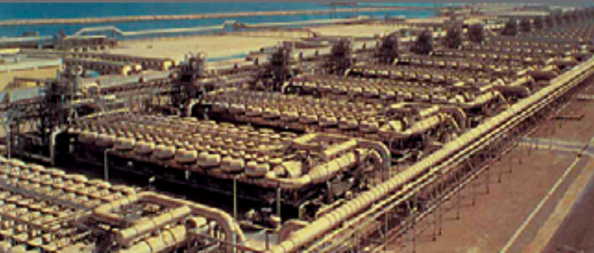
Figure 12. A few of the 40 units at Al-Jubail Phase 2, each 5 million GPD
