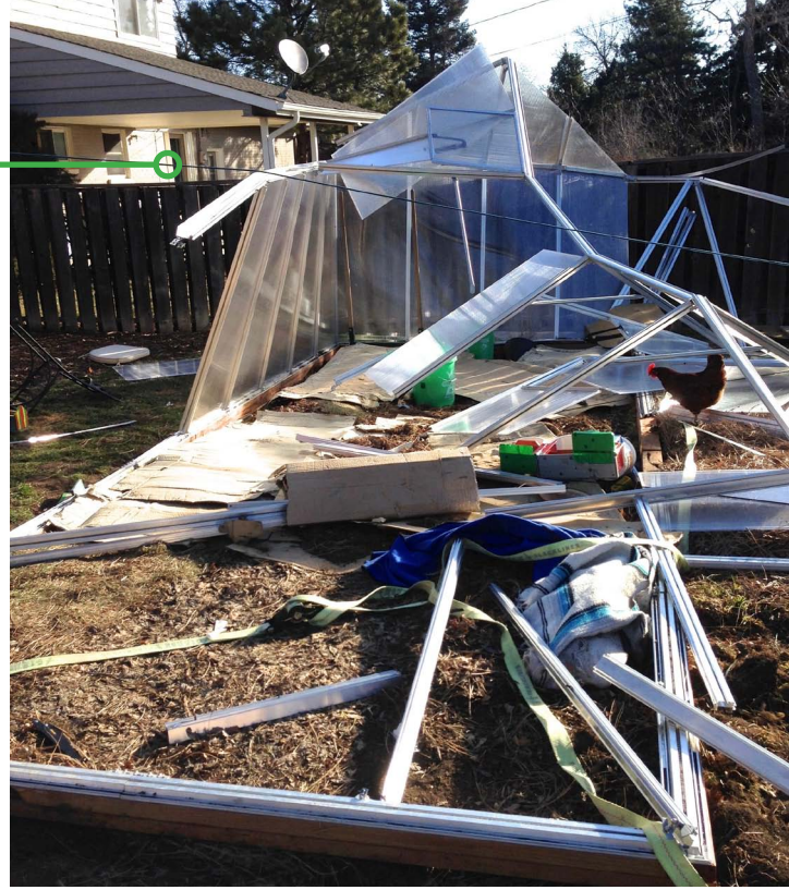
Above: A plastic kit greenhouse collapsed in a wind storm just a few weeks after it was put up. Standard greenhouses are usually not designed for the high snow or wind loads of many climates
