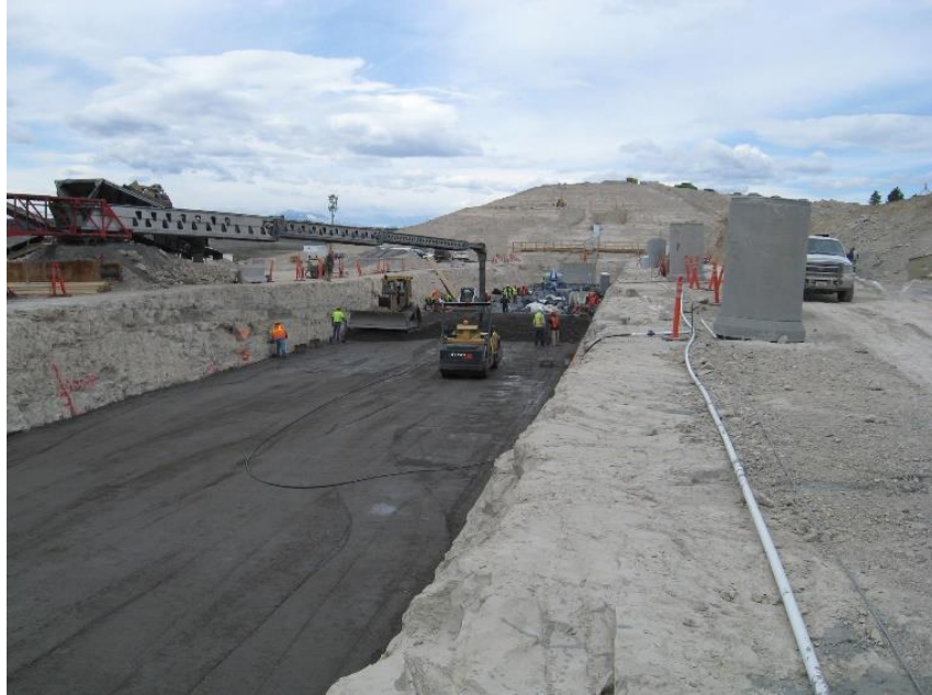
Figure 10-37. RCC placements in the cutoff.
