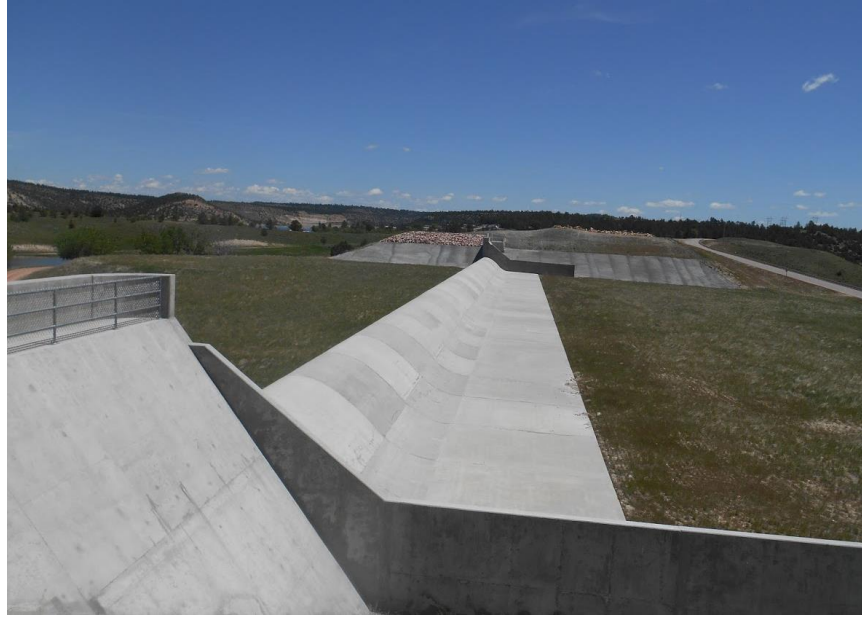
Figure 10-40. Completed auxiliary spillway.
