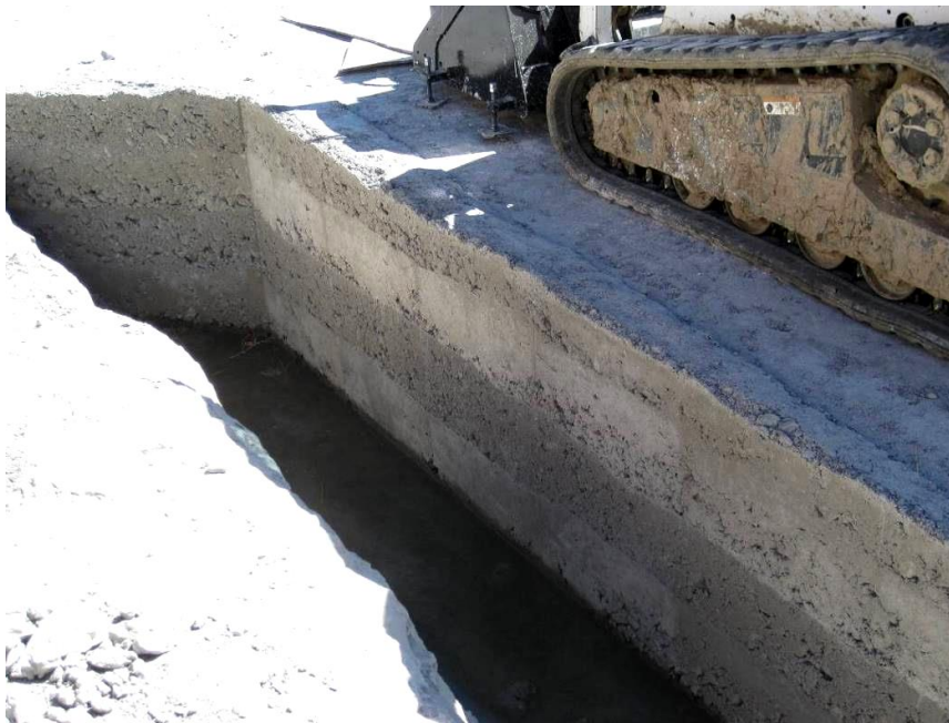
Figure 10-35. Placement of RCC test section demonstrating formed RCC without GERCC.
