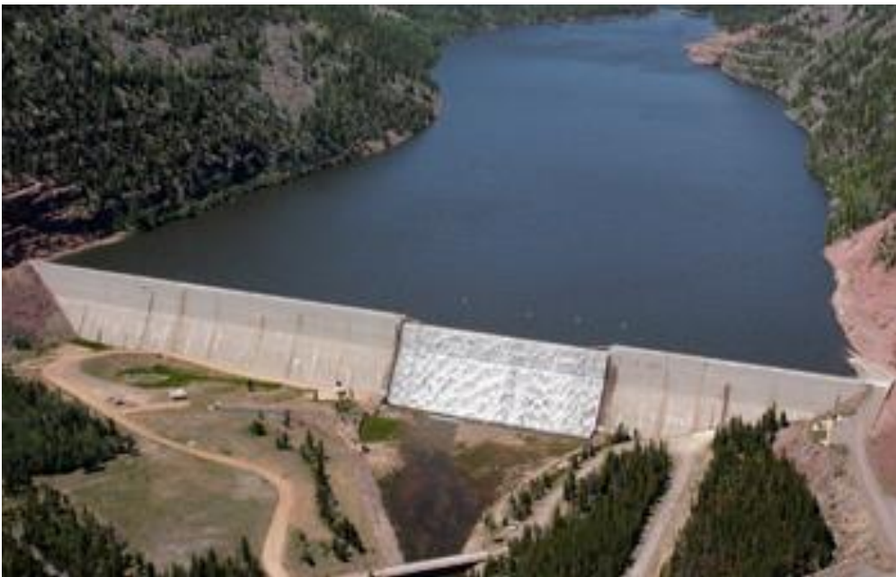
Figure 10-10. Aerial photograph of Upper Stillwater Dam with the stepped spillway operating.
