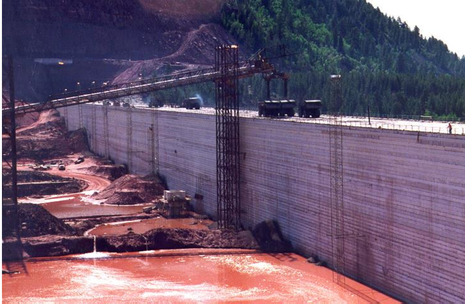
Figure 10-4. Photograph of the upstream face of Upper Stillwater Dam during construction.
