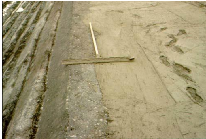
Figure 9-2. Bonding mortar used to improve sliding stability below the spillway crest.
