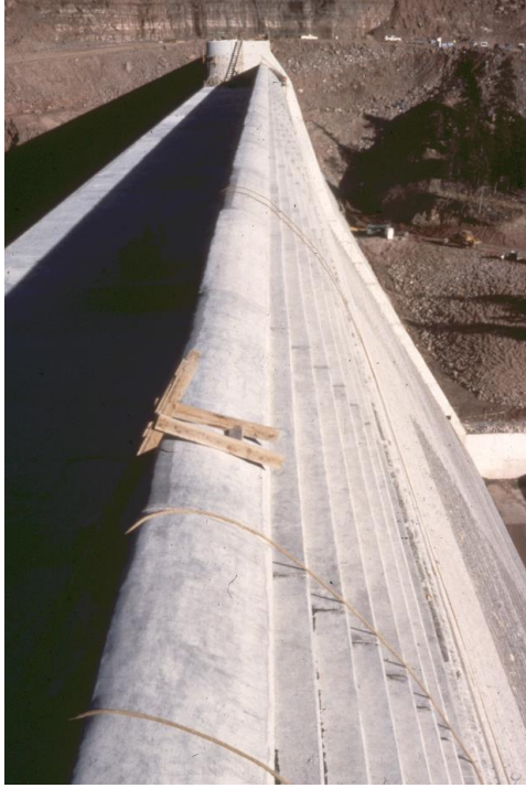
Figure 10-9. Spillway ogee crest under construction.
