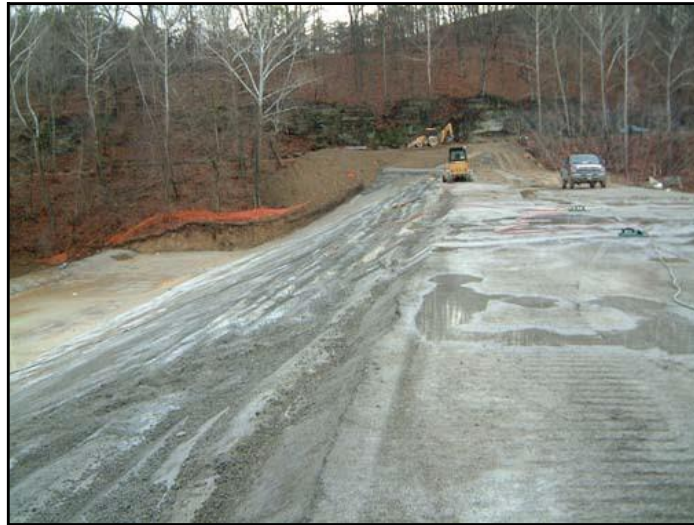
Figure 8-1. Overtopping protection at Vesuvius Dam during construction.
