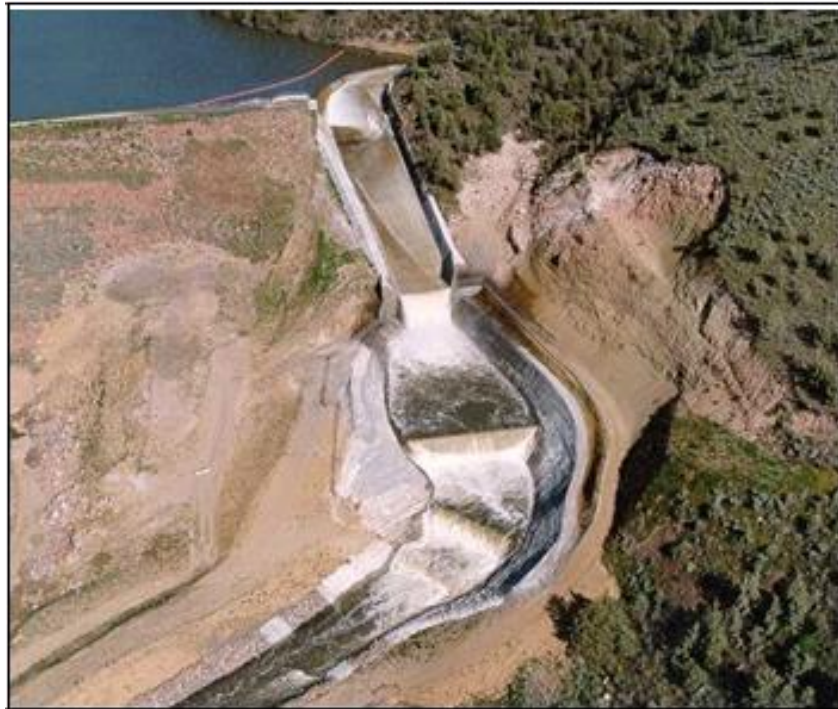
Figure 10-19. Aerial view of Ochoco spillway.
