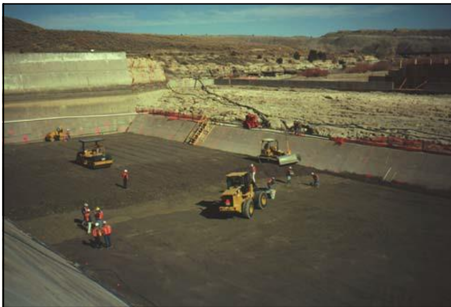
Figure 10-20. RCC construction in the stilling basin at Pueblo Dam.
