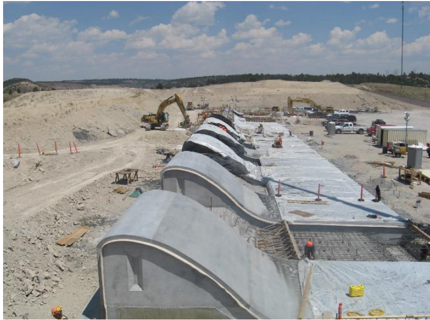
Figure 10-39. Conventional concrete placements for the ogee crest spillway.
