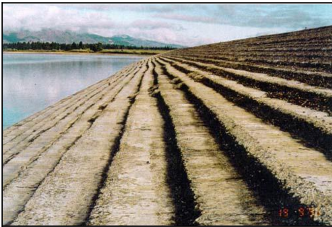
Figure 8-2. Upstream slope protection at Jackson Lake Dam, Wyoming.
