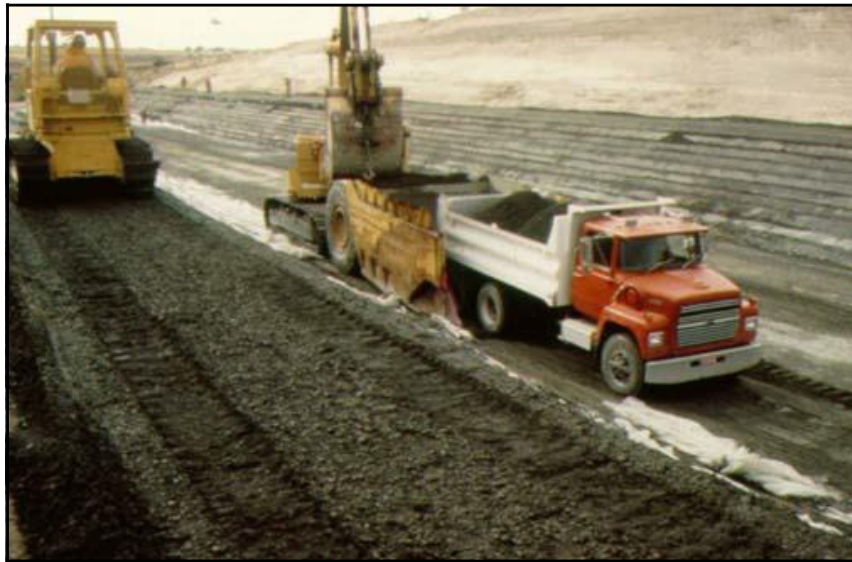
Figure 10-17. Placing RCC with a backhoe.
