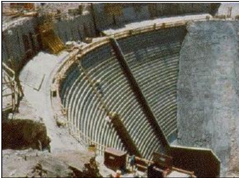
Figure 10-15. Downstream face of Santa Cruz Dam under construction.
