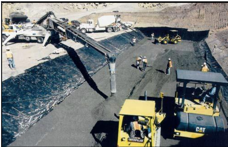
Figure 10-27. View of spillway stilling basin placement operations at Many Farms Dam.
