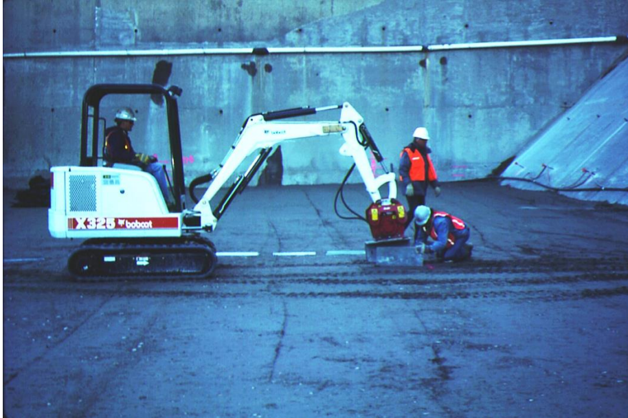
Figure 5-1. Installation of galvanized steel sheet at Pueblo Dam Modification.
