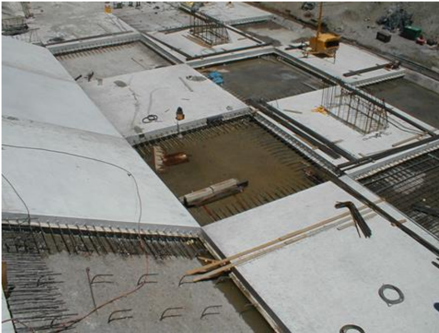
Figure 10-21. Conventional concrete overlay on the RCC stilling basin placements.
