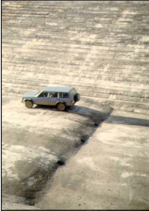
Figure 9-5. Small RCC weir in the Cold Springs spillway chute.
