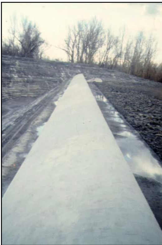
Figure 9-6. Conventional concrete ogee spillway crest placed over RCC.
