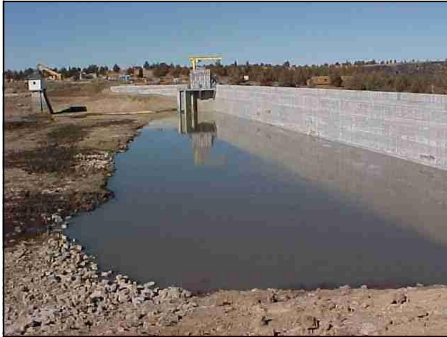
Figure 10-32. First filling of the completed Clear Lake Dam, an RCC gravity dam. New outlet works intake tower with control house and jib crane shown near left abutment. Original outlet works intake tower shown at left, on alignment of original embankment dam.
