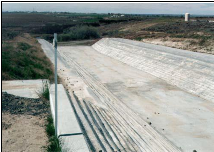
Figure 10-18. Completed RCC chute (Cold Springs Dam).
