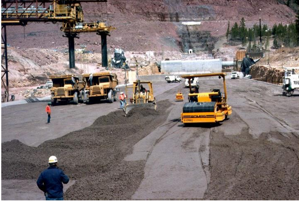
Figure 10-6. RCC placements showing spreading, compaction, and delivery systems.
