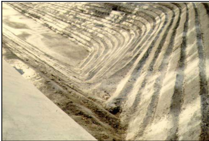
Figure 10-16. Tight turn radius at the upstream end.
