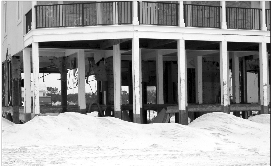
Figure 3. Successful breakaway wall performance
