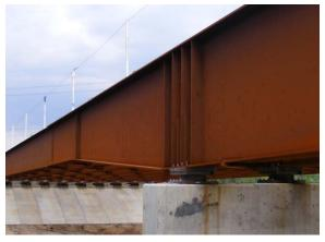
Figure 6: Girder Web Depth Transition at Pier 1, Looking Back Towards Abutment 1
