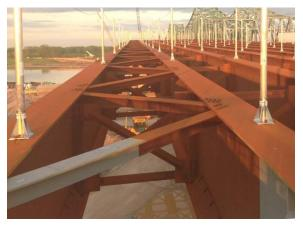
Figure 9: Top Flange Lateral Bracing
