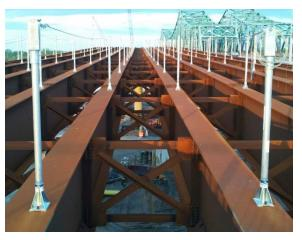
Figure 8: Typical Intermediate Cross-frames
