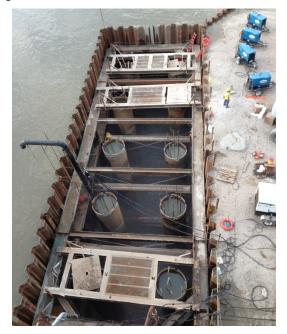
Figure 4: Pier 3 Drilled Shaft Construction
