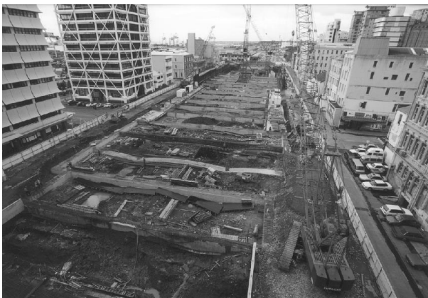
Photo 2 : View from West End. Roof beams cast on ground.
