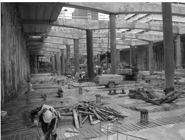
Photo 4 : View of secant pile walls and frames after excavation.
