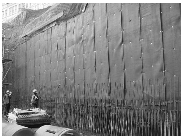
Photo 7 : Bentonite sheet nailed to rock surface prior to reinforcement placement
