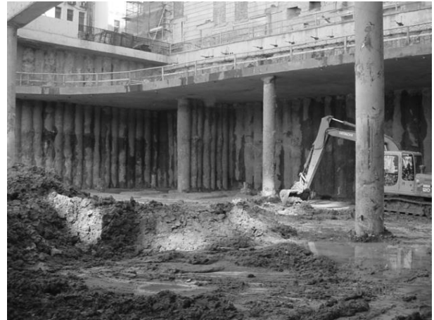
Photo 5 : View of walls and transfer slab after excavation
