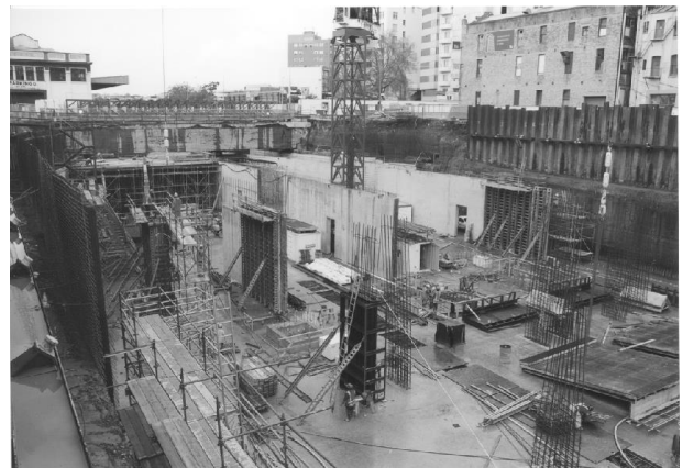
Photo 6 : East End. Bottom up construction within sheet piles
