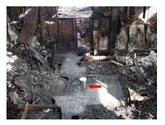
Figure 5 Debris field in wood frame construction
