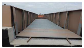
Figure 12: Placement of deck plates.
