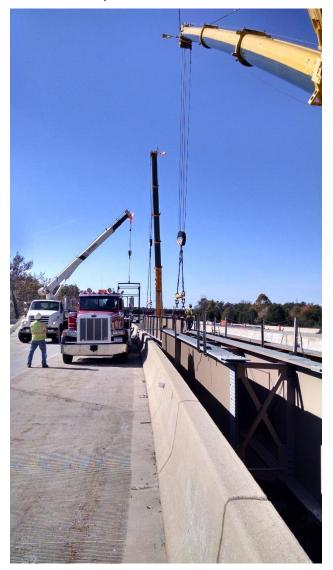
Figure 16: Broad Run girder erection.
