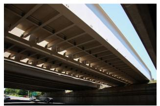
Figure 7: Completed steel framing.
