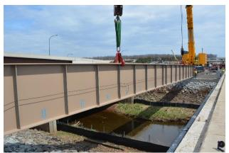
Figure 11: Girder erection over Horsepen Run.
