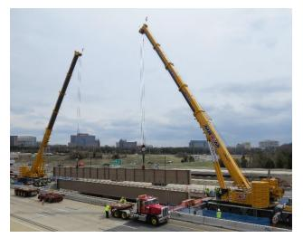
Figure 10: Girder delivery from adjacent bridge.
