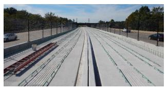
Figure 17: Finished concrete deck.
