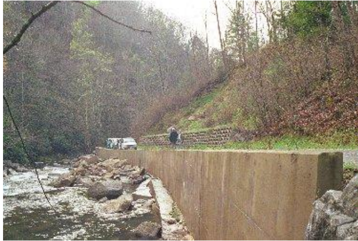
Figure. Photo of concrete retaining wall
