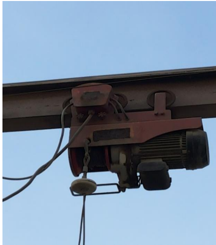
Fig. 16. Crane trolley mechanism
