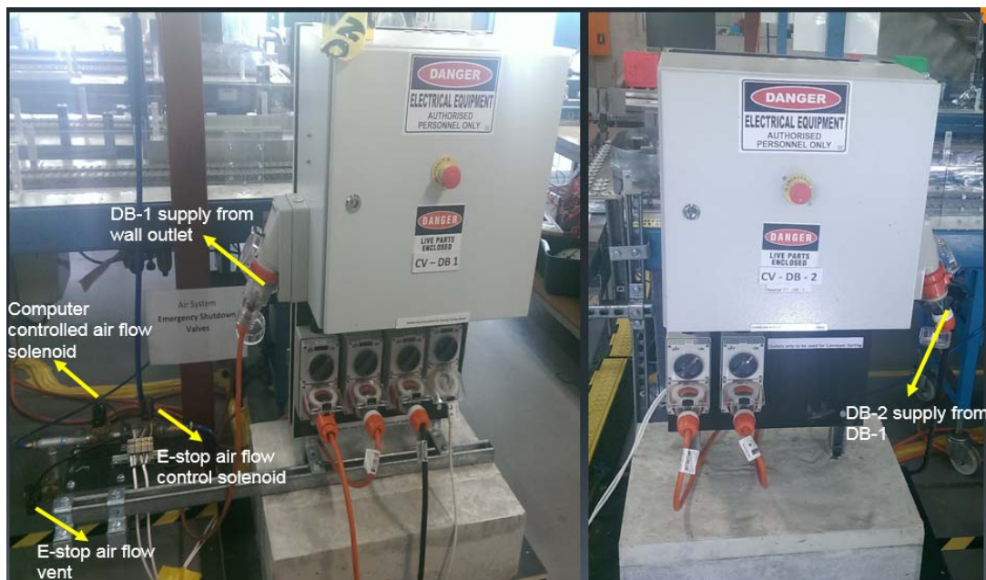
Figure 42: Distribution boards diagram
