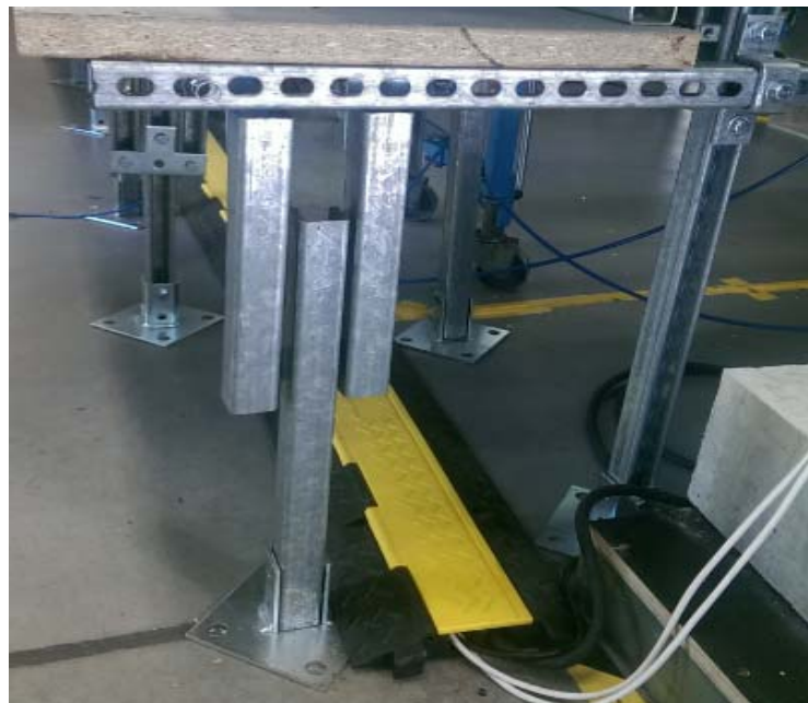
Figure 22: Base platform support made using strut channels
