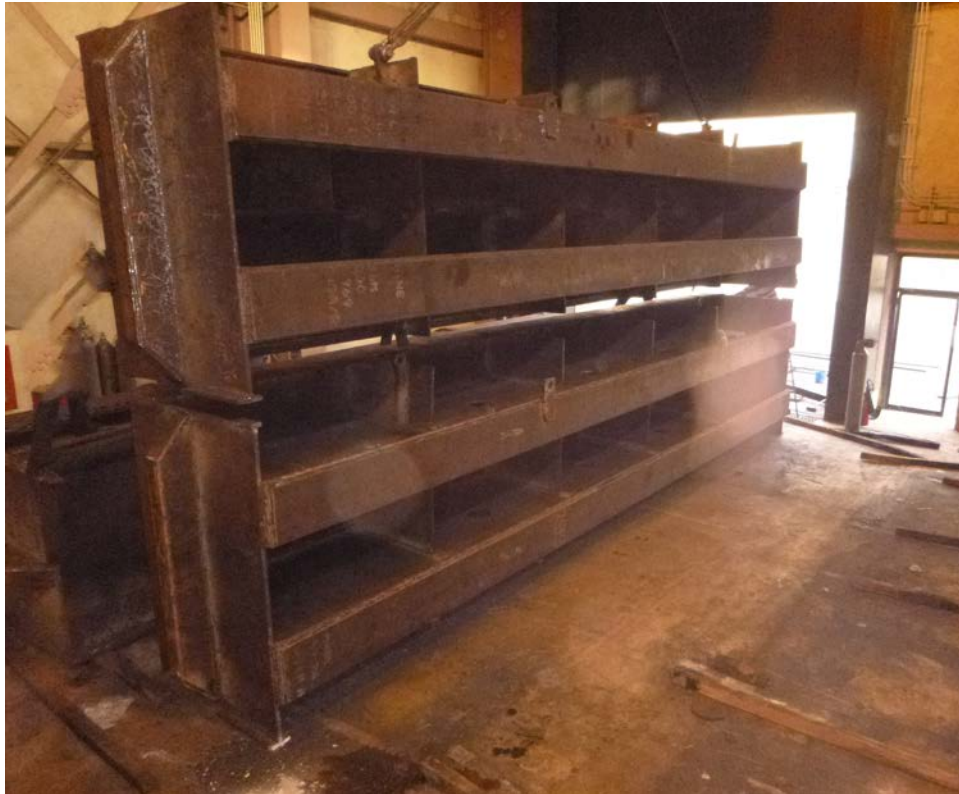
Figure 10. Fit-Up Test of Two Bulkhead Segments
