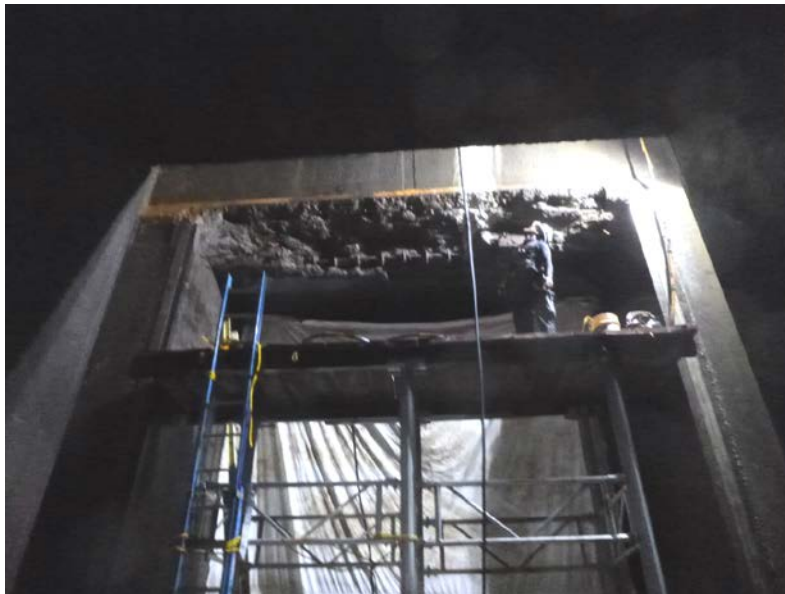
Figure 11. Preparing for Repair of the Damaged Lintel
