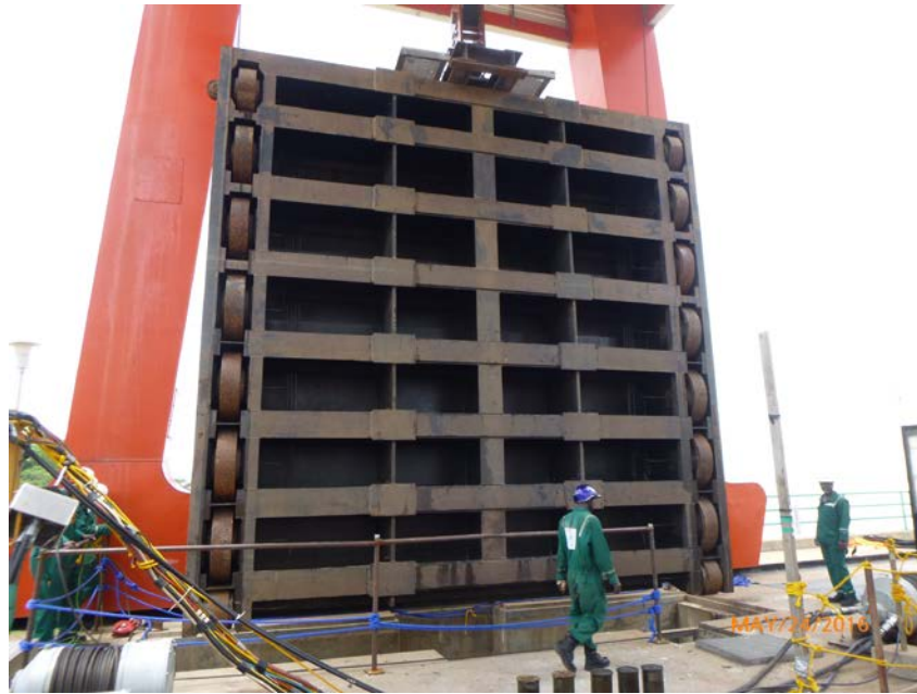
Figure 3. Downstream Side of Maintenance Gate Following Repair
