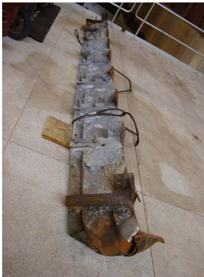
Figure 2. Lintel Seal Plate with Concrete Removed
