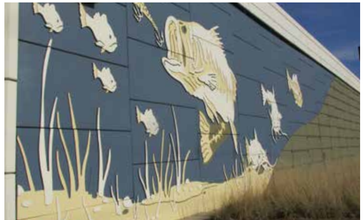
IH 35E Managed Lanes, Dallas & Denton, TX
