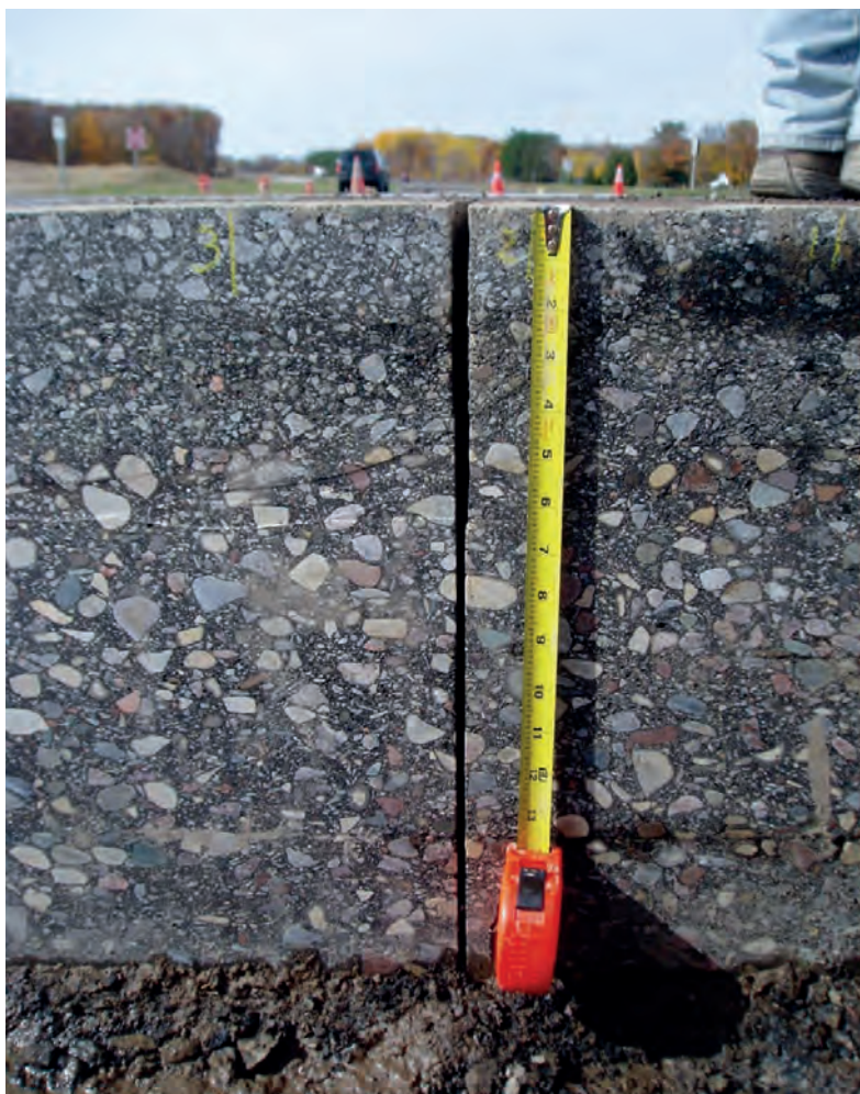
Figure 6-5. Different Asphalt Mixtures in the Pavement Structure
