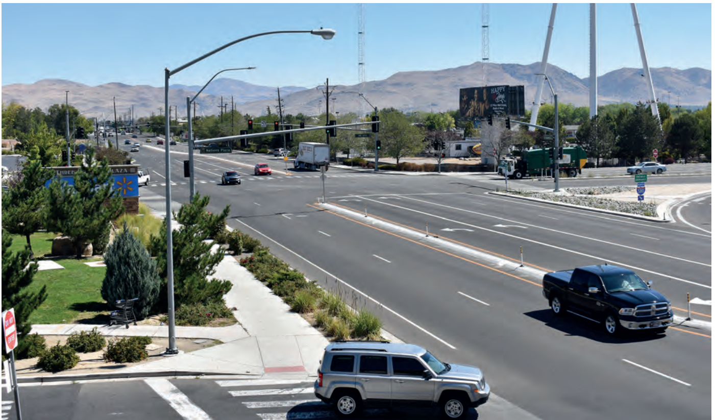
Because of heavy industrial truck traffic in the corridor, Glendale Avenue in Washoe County, Nevada, was reconstructed in 2018 with nearly 49,000 tons of a 19 mm NMAS mix. (Photo courtesy Granite Construction Co.)
