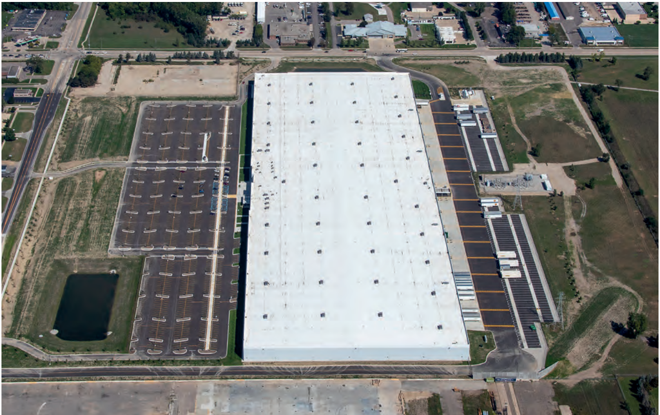
The heavy-duty lots at the Amazon Distribution Facility in Chesterfield Township, Michigan, made use of up to 40 percent RAP in the binder and surface layers. (Photo courtesy Cadillac Asphalt, a CRH Co.)
