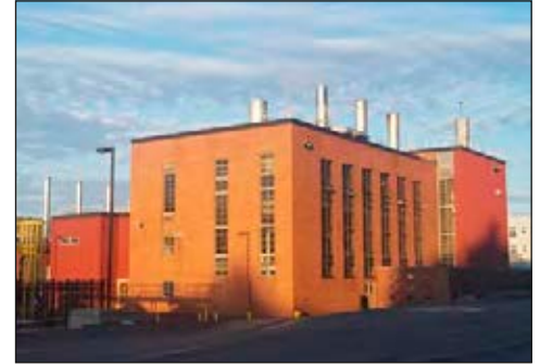
Michigan Tech Energy Management Central Heating Plant
