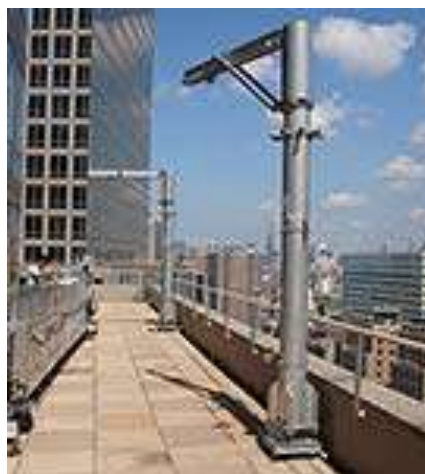
Figure 2 This photo shows how davits can be installed to provide a permanent suspension system.
