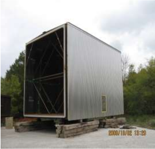
Figure 3- Insulated before raising into place
