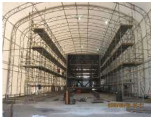
Figure 2 – This photo shows work inside the tent.
