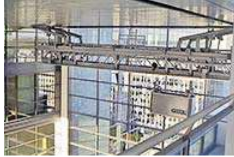
Figure 4 Gantry systems can be designed to maintain atriums and skylights.
