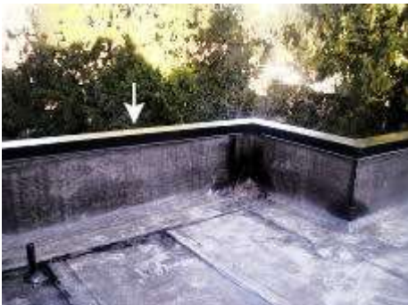
This photo shows a parapet wall around the roof edge
