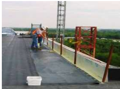
This photo shows a parapet wall installed on a bridge
