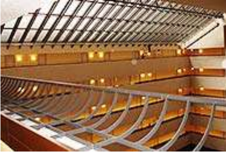
Figure 3 This photo shows how monorail systems can be installed along a building profile. They can be used to suspend work platforms.
