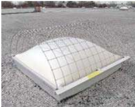
This photo shows a skylight guard
