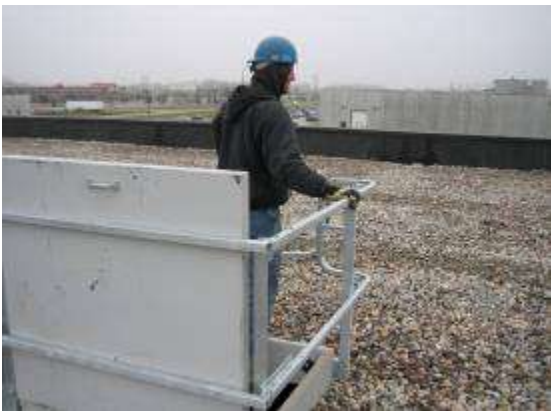
This photo shows a guardrail, swing gate, and grab bars
