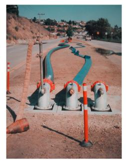
Figure 3. Flex Hose Attached to Manifold Outlets
