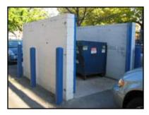
**Figure 2.13B** Not Appropriate: Don't enclose a trash enclosure in public view with concrete masonry.
