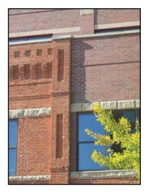
Figure 3.2A Appropriate: Keep original walls and build additions with compatible materials and details.
