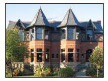
Figure 4.1.1A Appropriate: Do replace and use roof materials that are correct for style and
