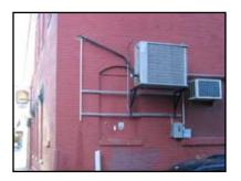
**Figure 2.12B** Not Appropriate: Utilities and/or mechanical equipment should not be seen from public right-of-way.
