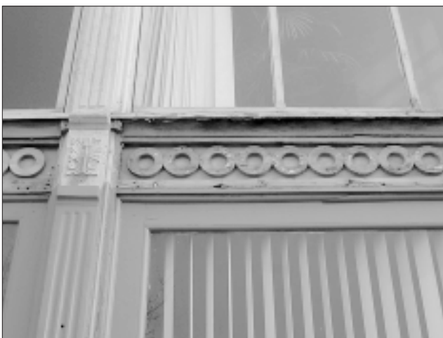
Protect wood features from deterioration.
