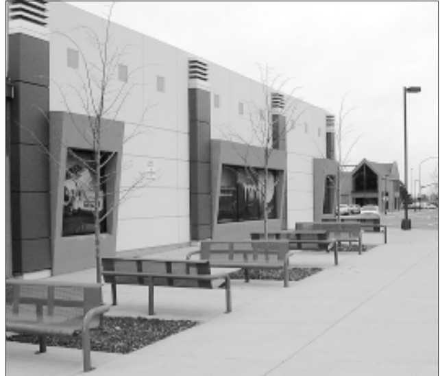
Consider using display cases on the ground floor where an active storefront is not a possibility. (Boulder, CO)
