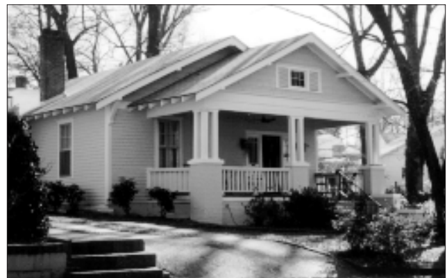
When replacing porch posts, use supports that are of adequate size. This porch reconstruction was based on neighboring houses of similar character and age. (Spartanburg, SC)
