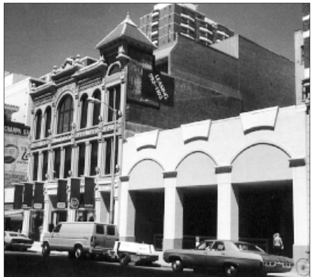
In the angle view above, two newer floors are visible. Note how in this building the addition cannot be seen when looking at the building straight on in the top photo. (Denver, CO)
