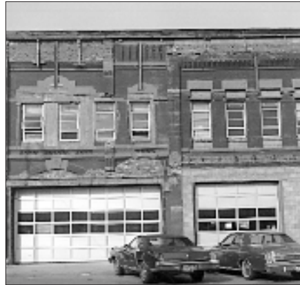
If a storefront is altered, restoring it to the original design is preferred. (Compare with the two photos of the same building below.)
