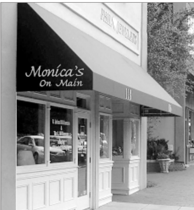
Alternative designs that are contemporary interpretations of traditional storefronts may be considered.
