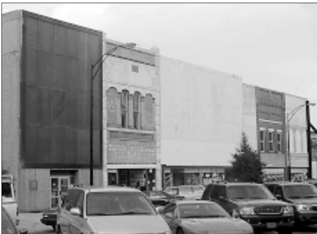
Some facades are covered, which obscures historic details.
