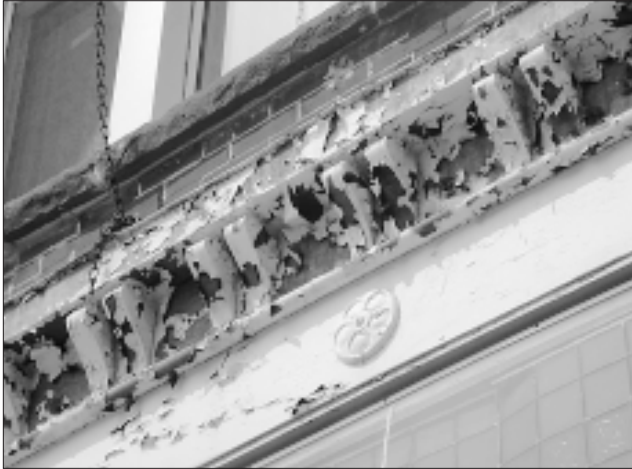
Maintain protective coatings, such as paint, on exposed metals.
