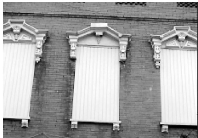
Enclosing an historic opening in a key character-defining facade is inappropriate, as is adding a new opening.
