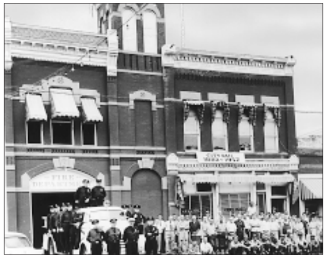
Using historic photographs can help in determining the original character. (Compare with below.)
