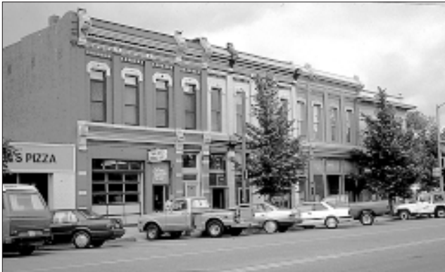
After rehabilitation, the row of buildings shown in the photograph above conveys a stronger sense of its historic character. Note that some old uses were retained, while other new uses were also introduced. Some noncontributing alterations were removed and storefronts reconstructed. One was retained, but was painted to minimize impacts. (Ft. Collins, CO)
