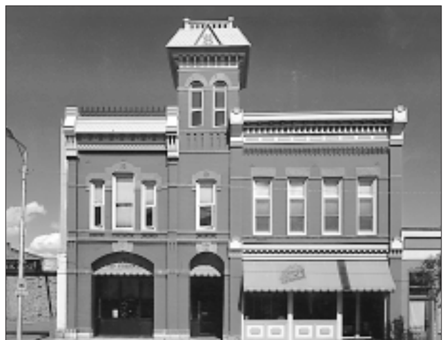
This rehabilitation preserves surviving details and reconstructs missing ones. (Ft. Collins, CO)
