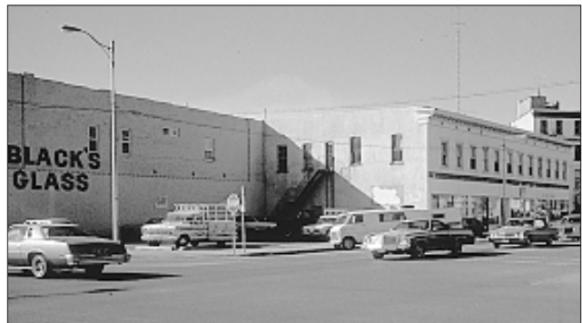
Before: New buildings should be compatible with the commercial buildings seen traditionally. Creative new design is especially encouraged that is compatible with the design goals of the district. Here, a parking lot awaits compatible infill. (See below.)
