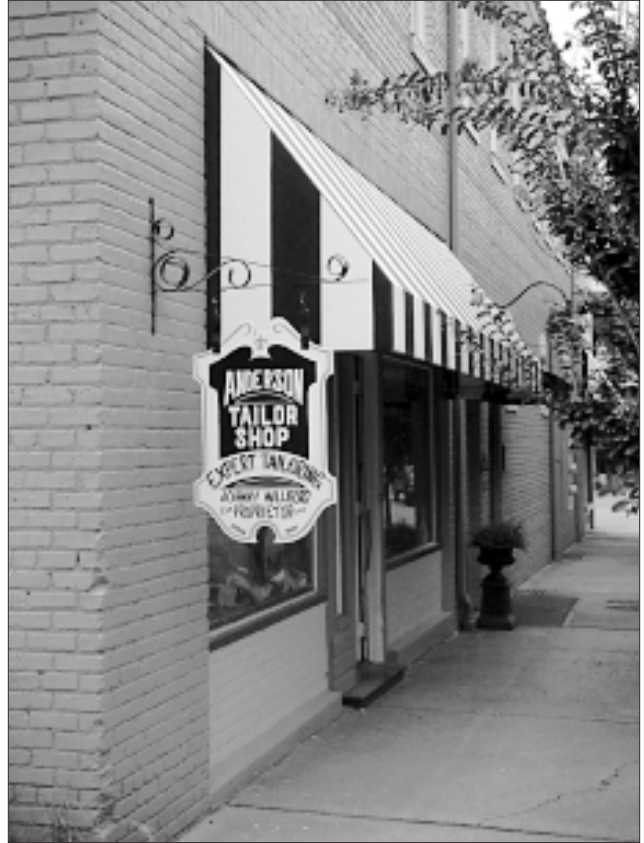
A larger projecting sign should be positioned at the corner of a building.
