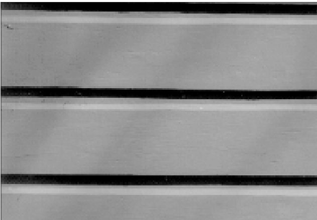
Maintain protective coatings to retard drying and ultraviolet damage. If the building was painted originally, it should remain painted.
