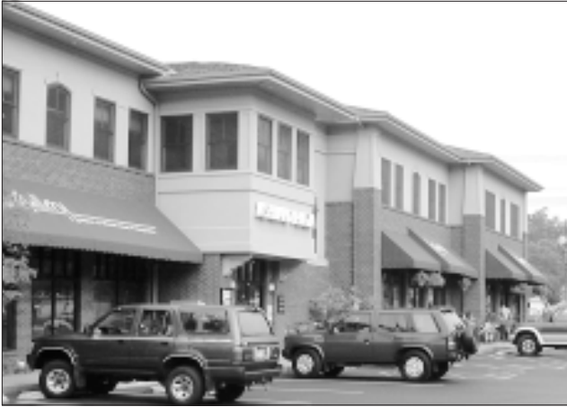
Consider dividing a larger building into “modules” that are similar in scale to buildings seen traditionally. (Bellingham, WA)
