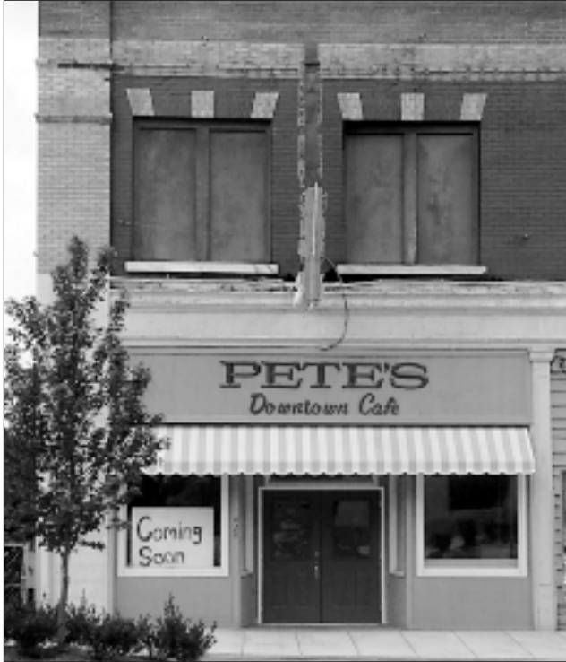
Restoring original openings which have been altered over time is encouraged.
