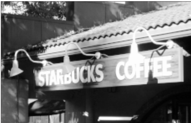
Lighting that is directed at a sign from an external, shielded lamp, is preferred.
