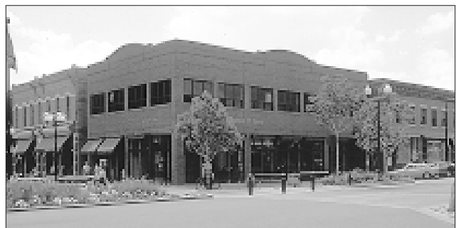
After: Simplified interpretations of traditional building elements, including a transparent first floor with display windows and an ornamental cornice, help this new building fit into its context.
