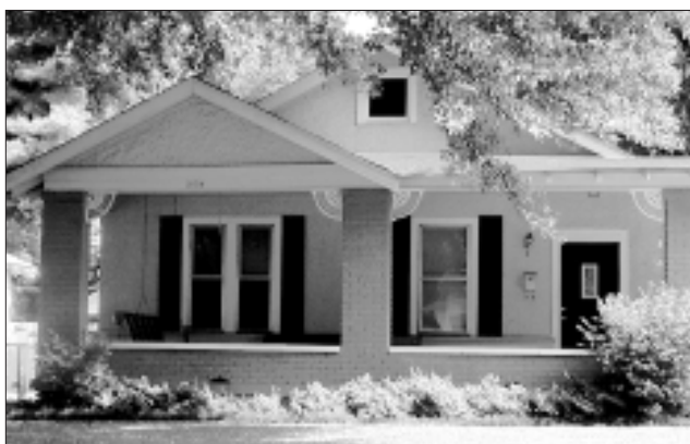
Dressing up a building with ornamentation out of character with the architectural style gives the building a false "history" it never had. This jigsaw ornamentation is out of character with the style and is inappropriate. (Memphis, TN)
