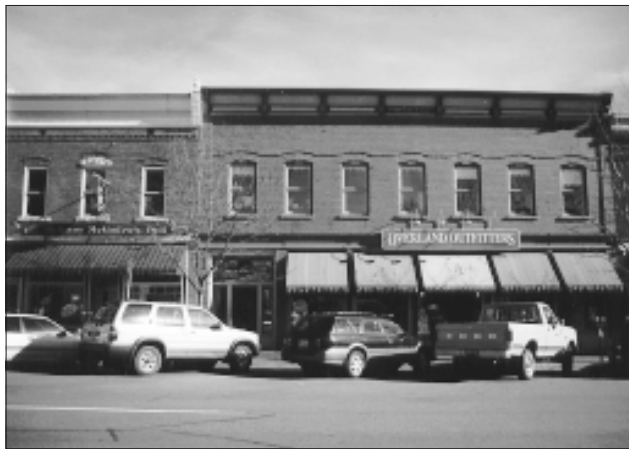
A sign band, awning and display window are traditional elements combined with a contemporary flavor.
