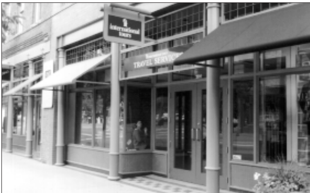
Contemporary interpretations of traditional building elements are encouraged. In this case, shed form awnings are stretched across rigid frames. Transom windows are expressed with a metal grill design.
