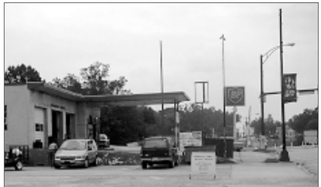
On the outer edges of downtown some buildings are set back from the street with places for automobiles in front. These appear in Area 2.
