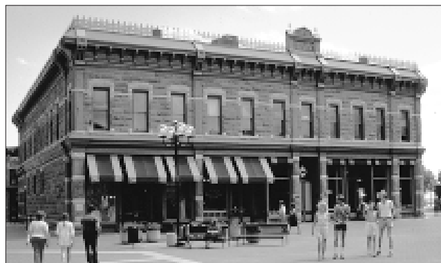
Storefront windows were reopened and upper-story windows were repaired. (Ft. Collins, CO)
