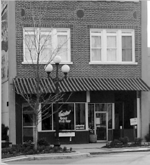
An awning compatible in material and construction to the style of the building is encouraged.
