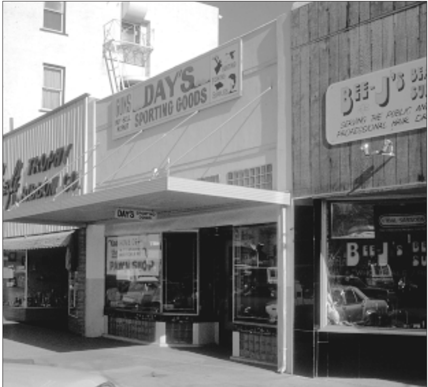
Years later, all original detail had been stripped from the building. (Compare with the photos above and below.)
