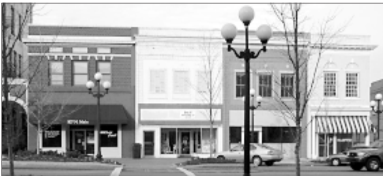
A building shall maintain the alignment of horizontal elements along the block.
