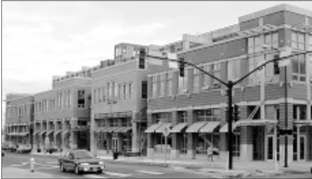
This single infill building is divided into smaller building modules that reflect traditional building widths. Upper floors step back from the front, thus maintaining the traditional two-story scale of the street.
