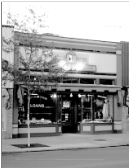
The same building (top) during renovation (left) and after renovation (above) exhibits the more classical features of commercial storefronts, including a painted cornice, kickplate and recessed entry. (Ft. Collins, CO)
