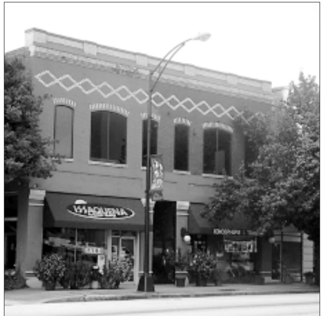
Usually between one and three stories, the vernacular commercial building is divided horizontally into two distinct bands. Some modest detail may exist.
