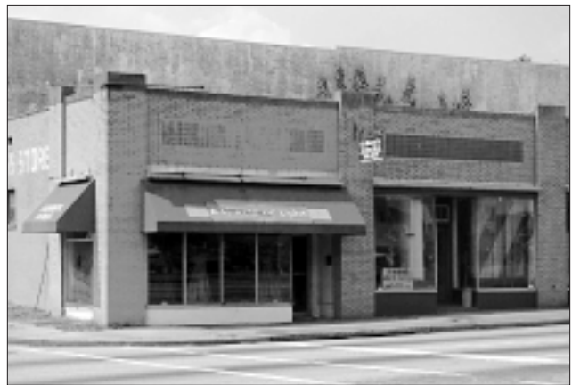
Many vernacular storefronts have simple display windows.
