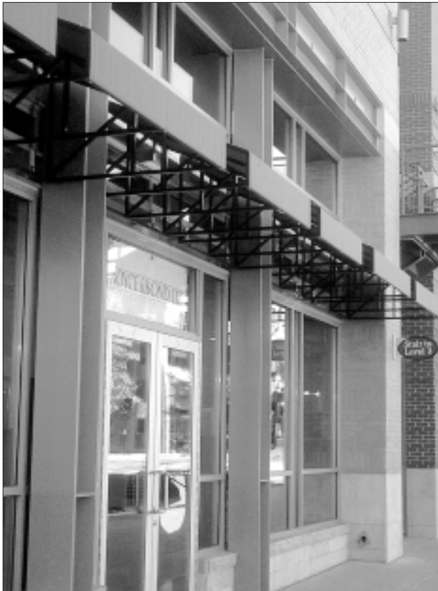
A new commercial storefront building should incorporate display windows, a transom window, a kickplate and recessed entry.
