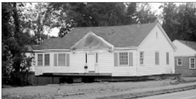
When use changes demand that structures be altered such that little or no use can be made of the original structure, consider moving the structure to a compatible location.
