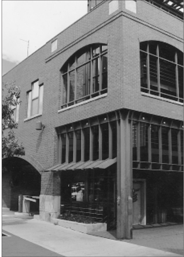
This parking structure incorporates a wrap of retail stores along the street edge. The storefronts are contemporary interpretations of the historic downtown context. (Boulder, CO)
