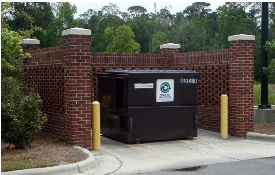
TYPICAL BRICK SCREEN WALL – PIERCED PATTERN
