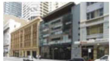
Case Study 09: Public building within a CBD historic context
