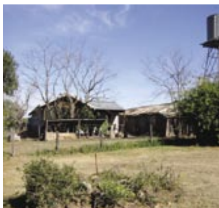
51 : The new house adjacent to the existing shed.
