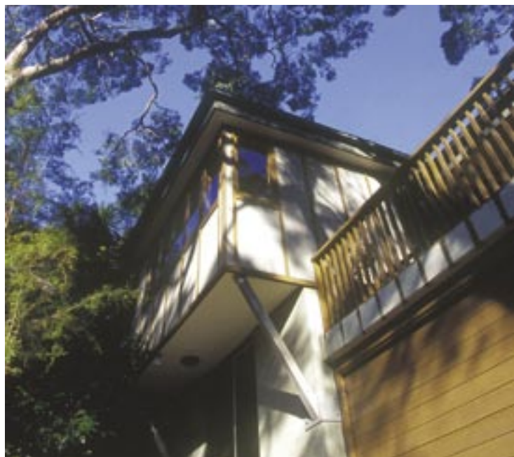
48 : The palette of materials and neutral colours makes the houses relate to, but differ subtly from, the existing house.
