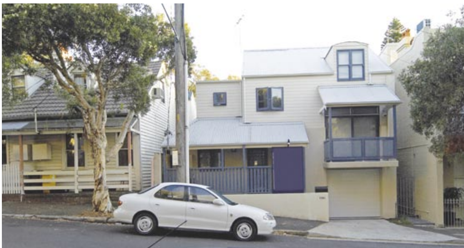
41 : The new two-storey house makes the transition from single-storey to two-storey and accommodates off-street parking without the garage becoming a dominant element.
