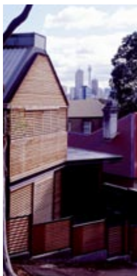
37 : The new two-storey section of the house with timber cladding.
