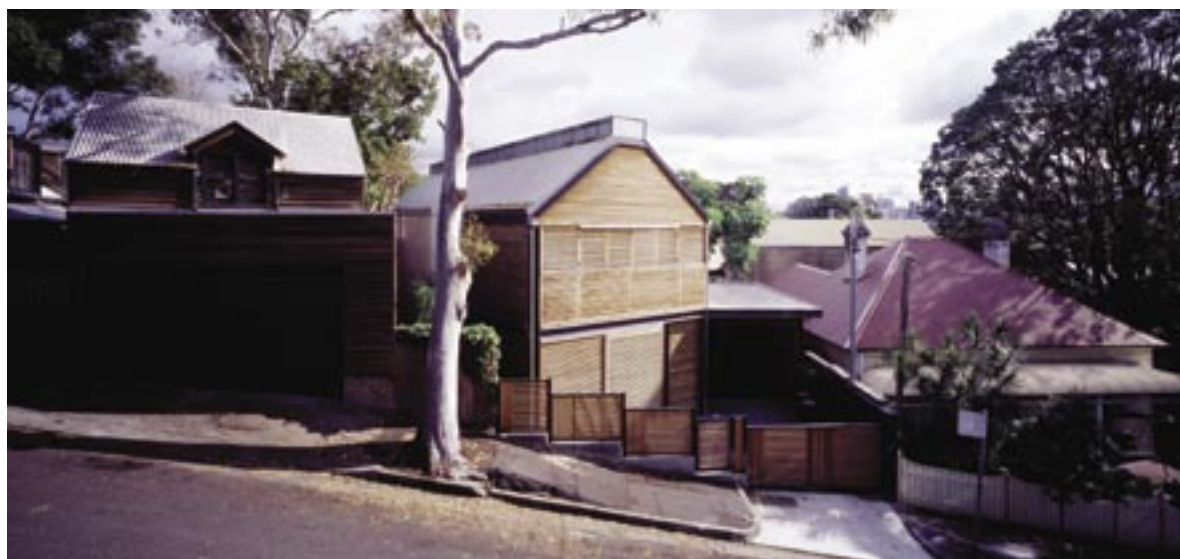
38 : The new house in context with its two-storey and single-storey neighbours.
