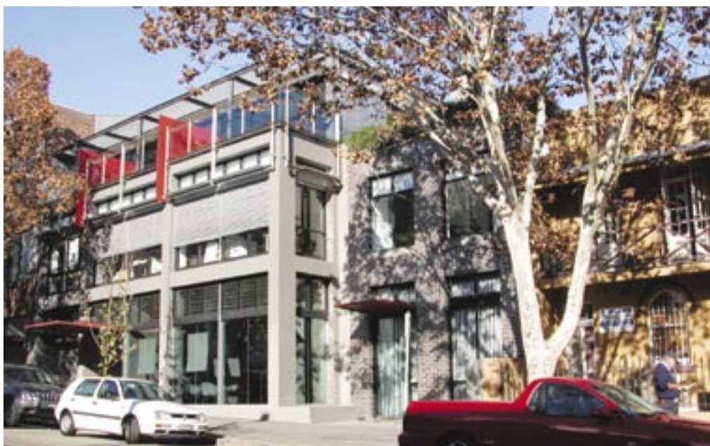
64 : The building site between existing terraces and a nondescript warehouse. It provides a transition between these but responds to the industrialised buildings of the area.
