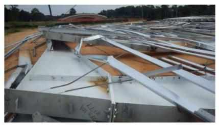
Photograph 8: Diagonal rod bracing is installed in the west sidewall, between the third and fourth rigid frame columns from the north side of the building.
