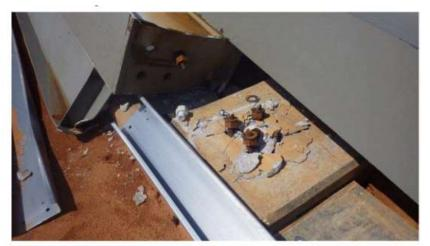
Photograph 18: The majority of the anchor bolts are sheared, either above or below the base plate of the rigid frame columns.
