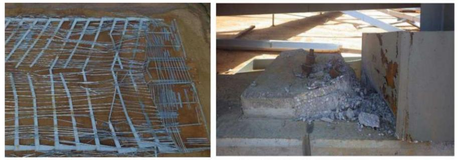
Photograph 19: The majority of the concrete pile caps are cracked.
