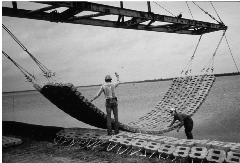
Figure 7.3—Close-up of spreader bar and ACB mat.
