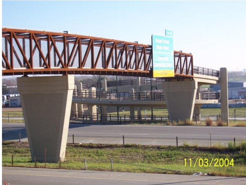
Figure 7. Example of pedestrian truss bridge utilizing weathering steel members.
