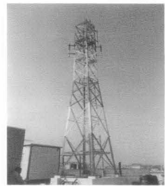
Figure 3. Self Supporting Tower.
