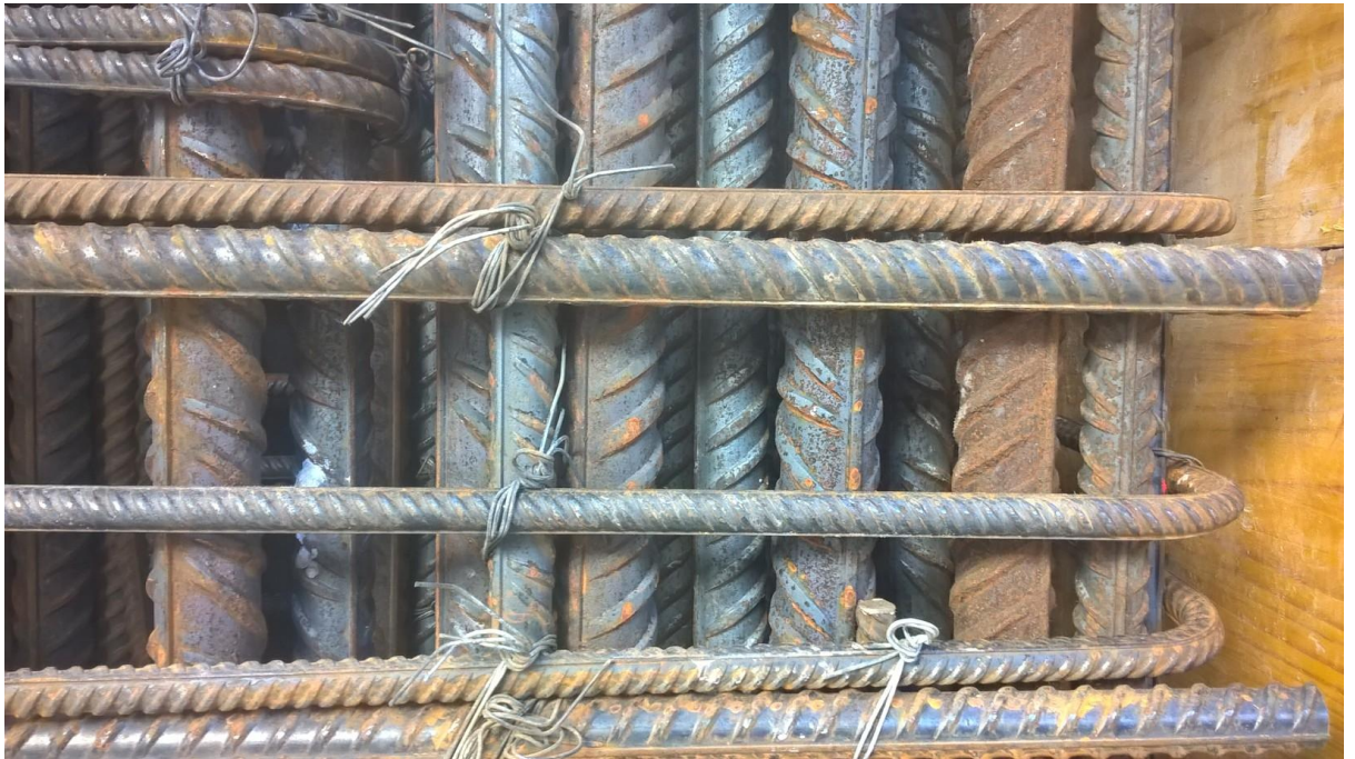
Figure 5. Dense reinforcement installed at construction site. (Sweco Rakennetekniikka Oy. 2017)
