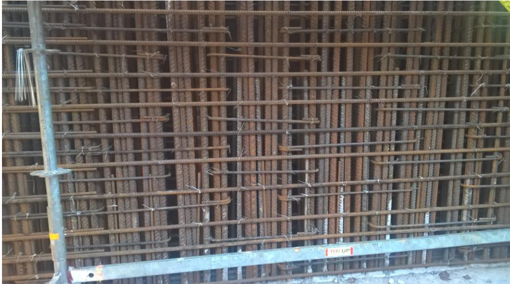
Figure 8. Installed reinforcement. (15.)
