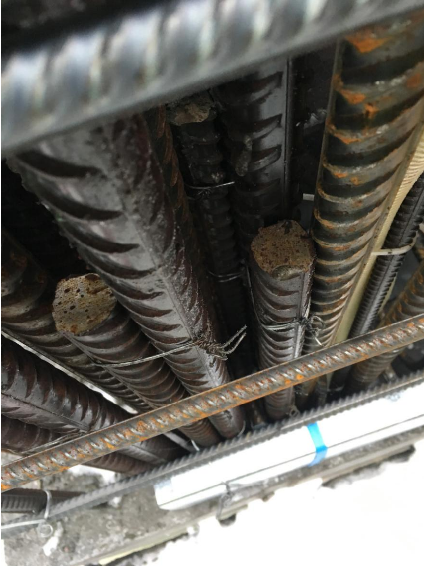
Figure 13. Installed rebars at construction site.
