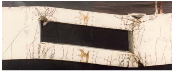
Fig. 10. Ductile failure of a beam under combined bending and shear.
