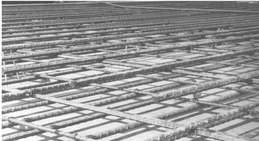
Figure: sample picture of placement of reinforcement.
