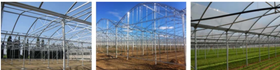
Figure 7: Galvanized steel structures images.
