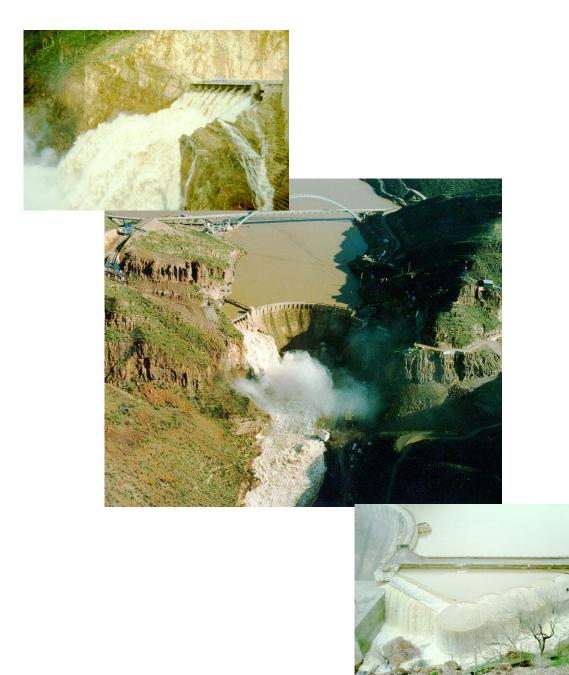
Figure 2.2.1-1. Example: Flood event (estimated inflow peak of about 89,600 cubic feet per second [ft<sup>3</sup>/s]) occurred during construction of a dam safety modification in 1993 (center photograph). This resulted in the existing right abutment service spillway passing about 41,600 ft<sup>3</sup>/s (upper left photograph), and the left abutment cellular cofferdam being overtopped, but failure did not occur (lower right photograph). Theodore Roosevelt Dam, Arizona.
