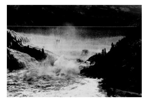
Figure 2.2.1-2. Example: Flood event (estimated inflow peak of about 60,000 ft<sup>3</sup>/s) occurred in 1964. This resulted in the discharge capacity of the service spillway being exceeded and the gravity arch dam being overtopped by about 3 feet for 20 hours. Gate closures and unsuccessful operations contributed to the overtopping. The dam crest and foundation were modified in 1982 to safely accommodate overtopping for floods greater than the 100-year event. Gibson Dam, Montana.
