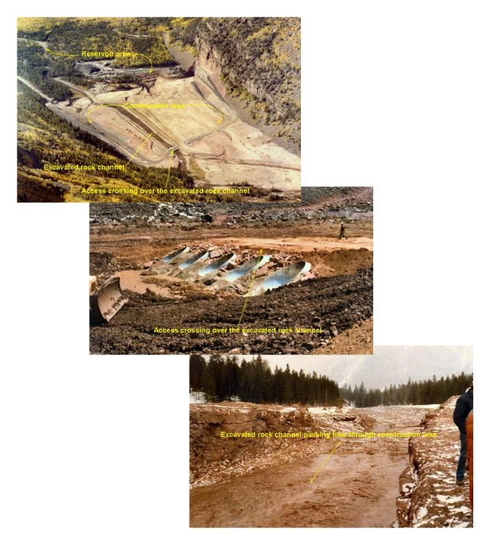
Figures 2.5.1-3. Example: Construction diversion method. Upper photograph: excavated rock channel without cofferdam through the construction site. Center photograph: access over the excavated rock channel. Lower photograph: close-up of the excavated rock channel. Upper Stillwater Dam site, Utah.
