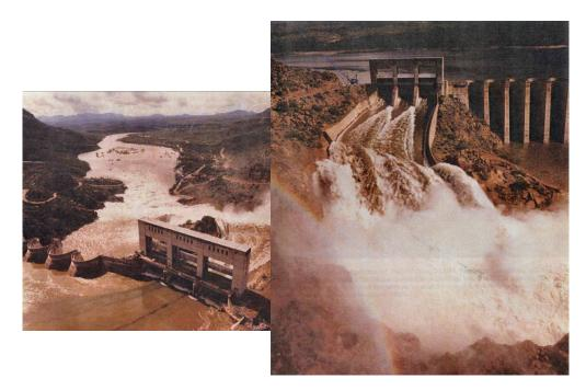
Figure 2.2.1-4. Example: Flood event (estimated inflow peak of about 100,000 ft<sup>3</sup>/s) occurred during construction of a dam safety modification in 1995, which swept away cross-river access to construction site. Bartlett Dam, Arizona.
