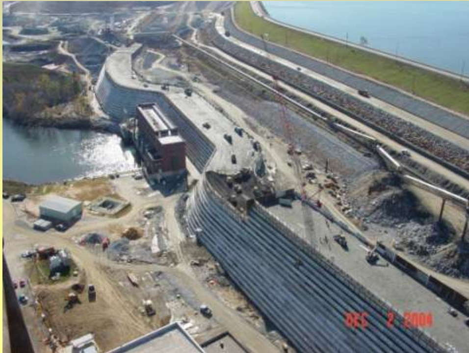
Newly constructed concrete backup dam, Lake Murray, SC
