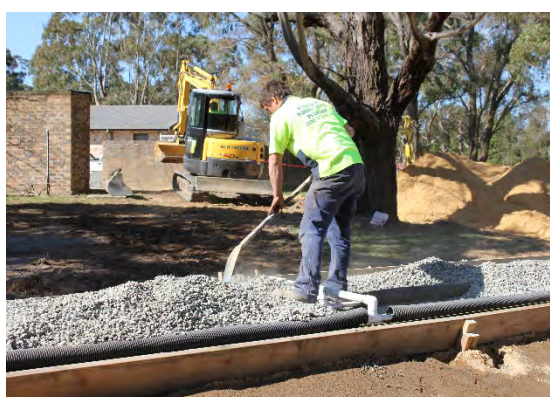
Figure 9.5 Gravel over inlet manifold
