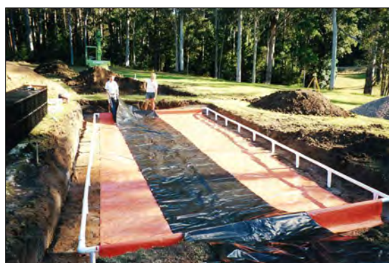
Figure 8.4 Construction membrane
