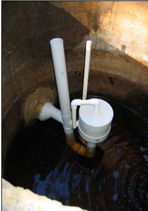
Figure 10.3 Dosing siphon (Arris Wastewater Clinic)
