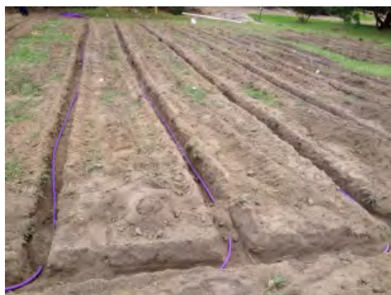
Figure 13.1 A subsurface irrigation system under construction (Warrnambool City Council)
