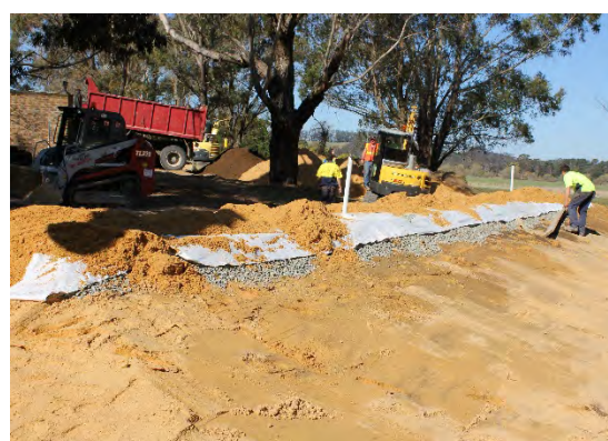
Figure 9.6 Sand on top of geotextile fabric
