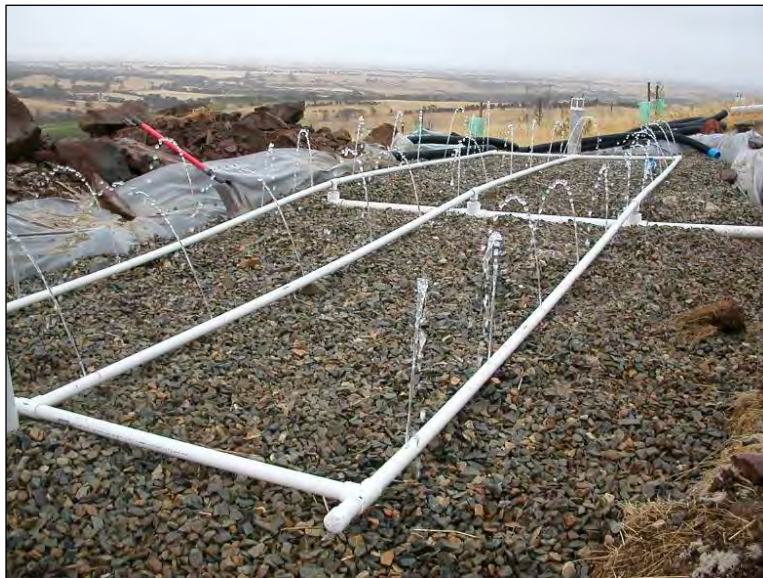
Figure 11.3 Pressure testing the distribution laterals for even distribution of effluent (Source: D Stafford)
