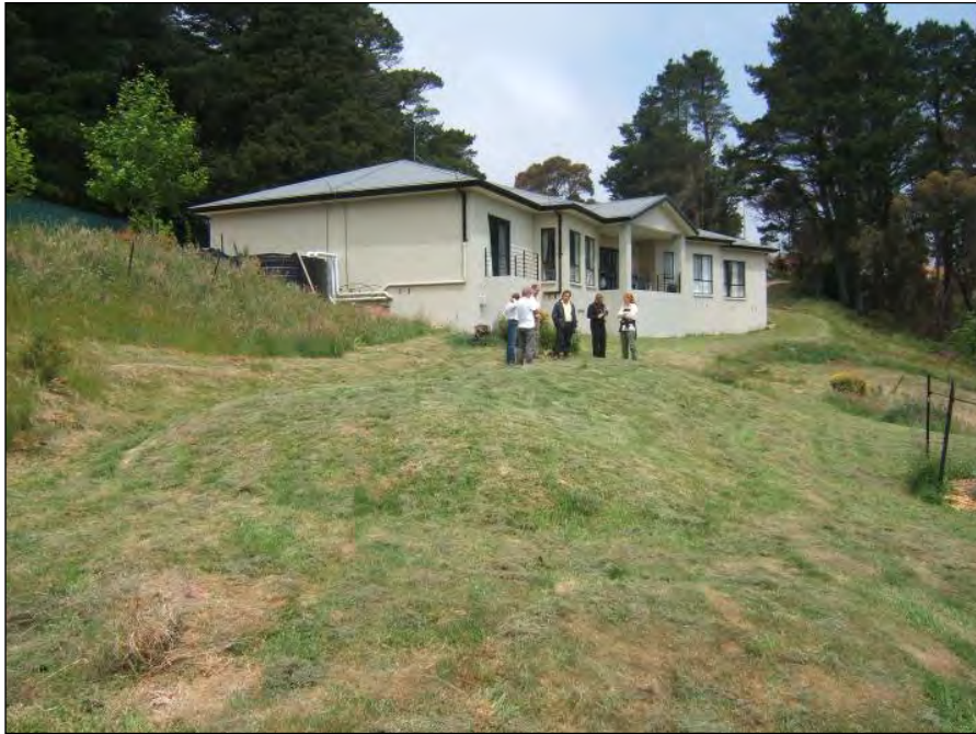
Figure 8.9 Amended soil mound constructed on sloping site
