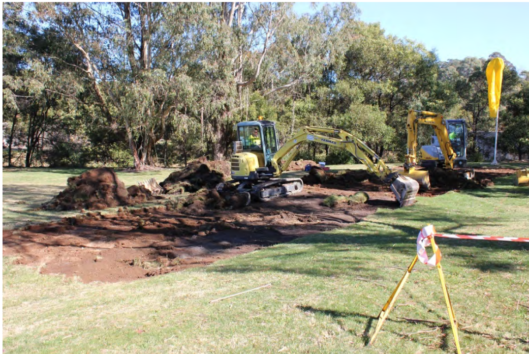
Figure 9.2 Excavation/preparation of base of mound
