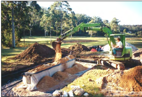
Figure 8.6 Backfilling with amended soil
