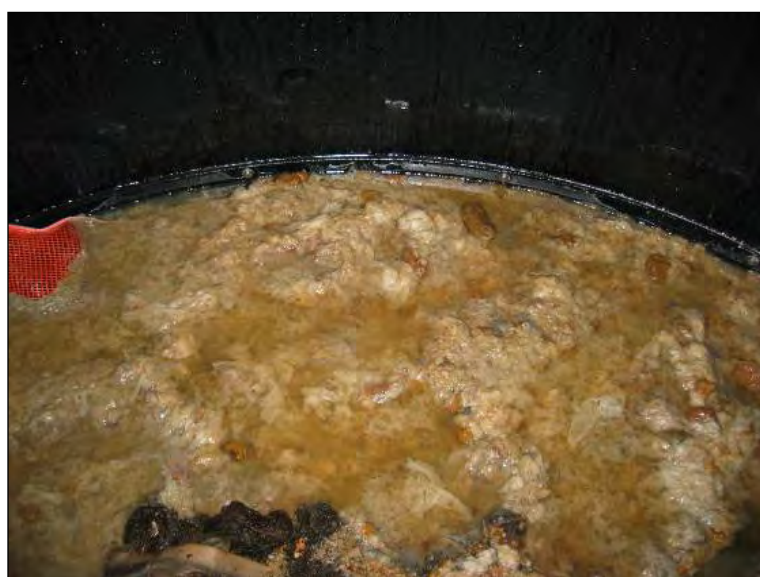
Figure 5.9 A flooded system due to pump failure
