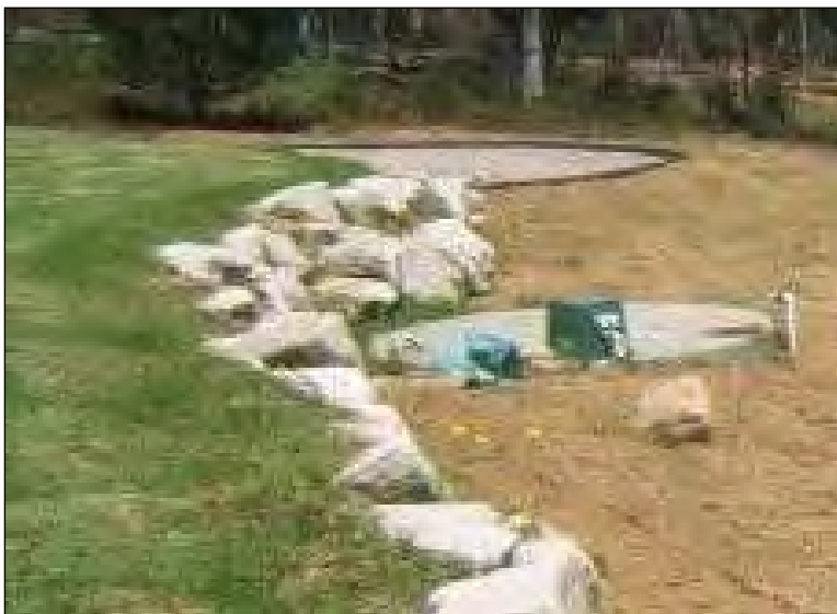
Figure 13.10 One of the new zones at the rear of the property established upslope of the aerated wastewater treatment system on imported soil
