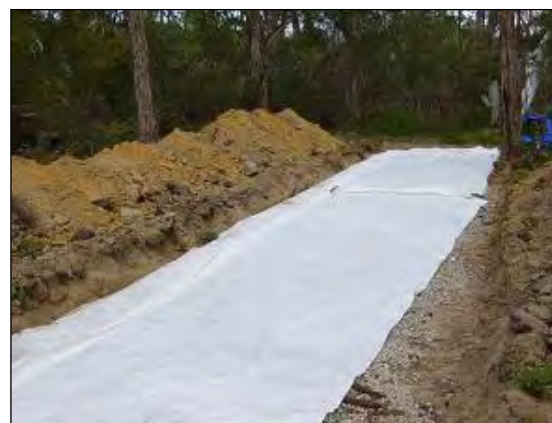
Figure 10.19 Adding the second geotextile fabric layer
