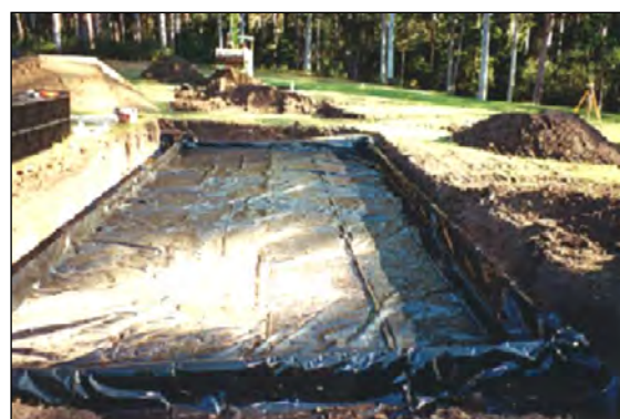
Figure 8.5 Lining with an impervious liner
