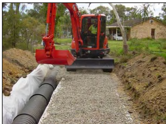
Figures 10.18 Backfilling gravel layer
