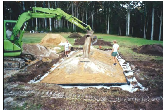
Figure 8.7 Final shaping of cell mound
