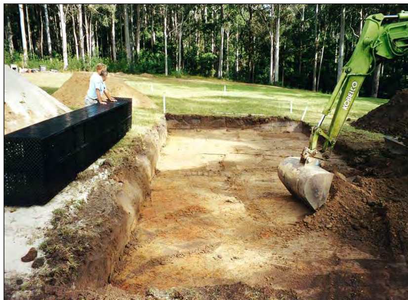
Figure 8.3 Excavation/preparation of base of mound (Figures 8.3-8.7 Ecomax, 2001)
