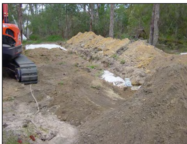
Figure 10.20 Backfilling and the inspection ports
