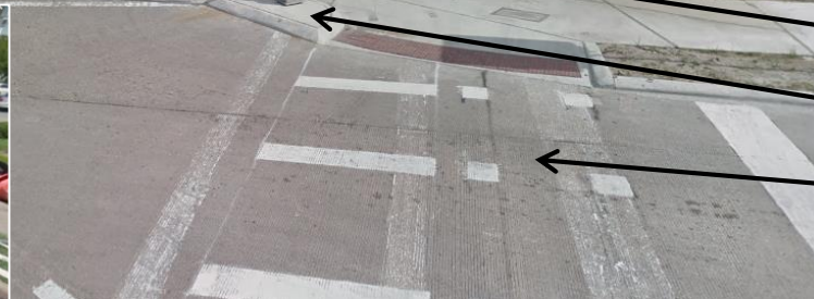
Pedestrian Crosswalk Bicycle Crosswalk
