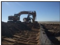
Construct Heavy Sniper Range 18
