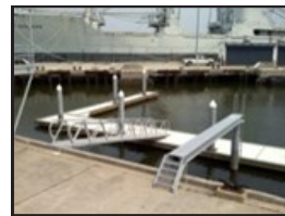
Design-Build Maritime Practical Applications Training Facility
