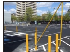
Remove & Install New Parking Lot & Security Fencing
