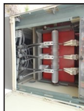
Repair Base Electrical Feed
