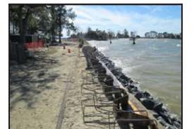
Repair Short Stay Wall Rec Area Lake Wall
