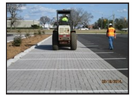
Repair Parking Lot
