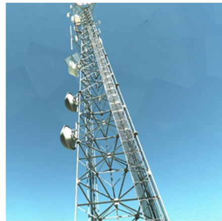
Figure 3 Lattice Tower transparent.
