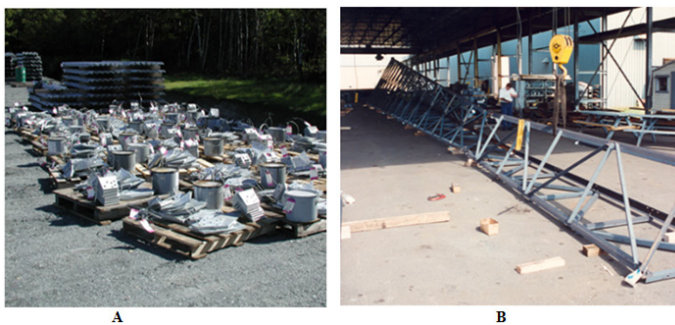
Figure 1 (A) Lattice tower easy transport and (B) on-site assembly.
