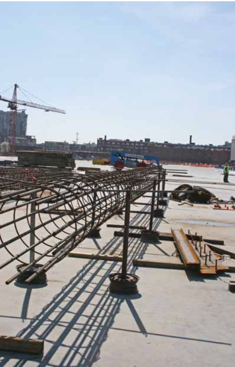
Fig. 4: Horses are used to support a column cage during fabrication
