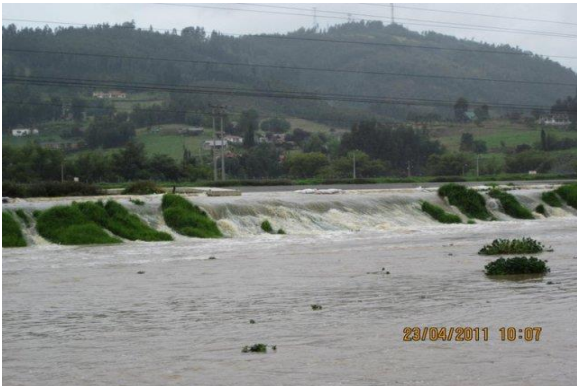
2011 Flooding Conditions Downstream La Copa Dam
