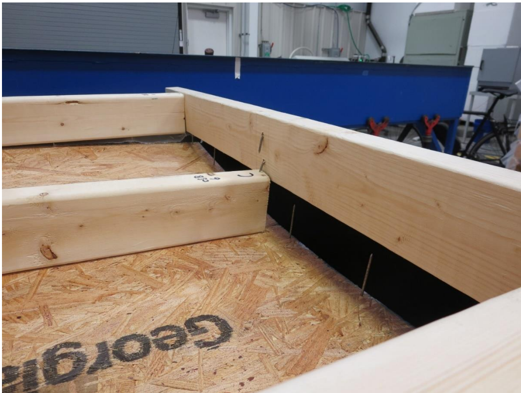
Figure 5 - 2. Failure of wall panel by nail withdrawal from along the bottom wall plate
