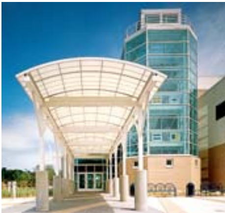
Mona Shores High School, Mona Shores, MI URS Greiner, Architects
