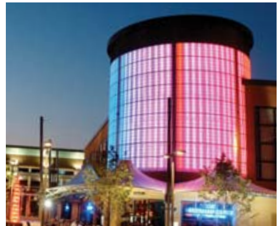
Merry Hill Shopping Centre, Brierley Hill INC Design Associates, Architects
