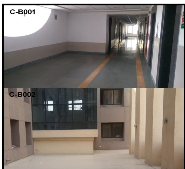
Figure 7. CCTV for Fire Detection at RGIPT
