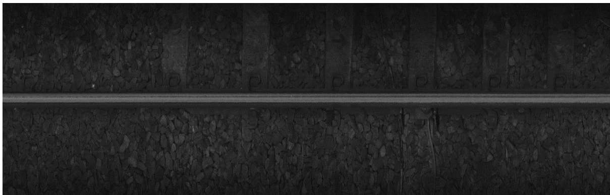
Figure 38: Sample image from data set containing completely obscured sleepers and fasteners (leftmost sleepers)
